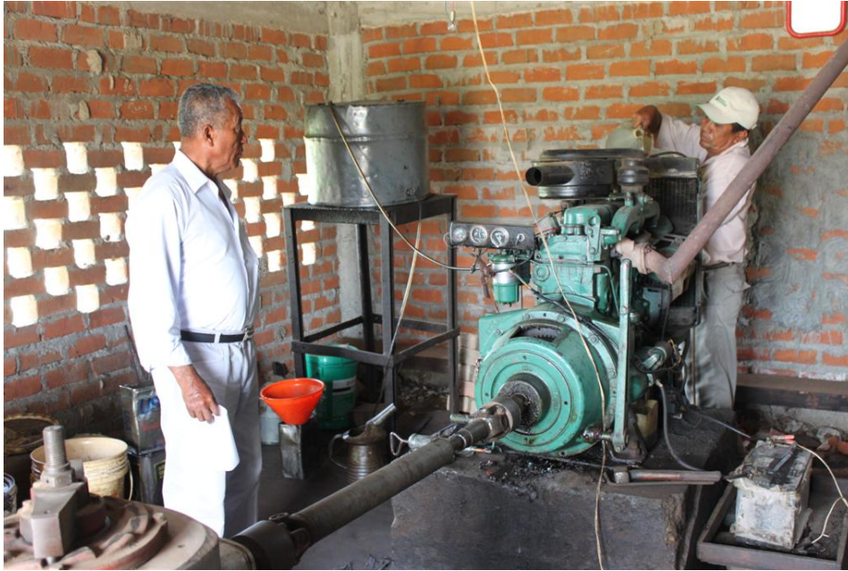
Figure 26. The old motor powering Yapatera's well.
