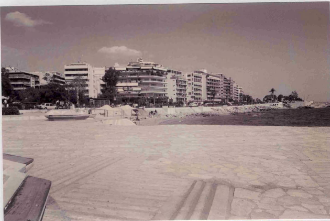
Photograph 5.30 'PHLISVOS'. THE PIER
