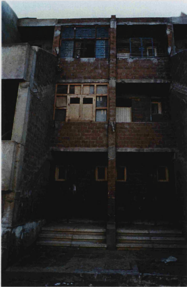
Entrance to a block of flats, Neighbourhood 5
