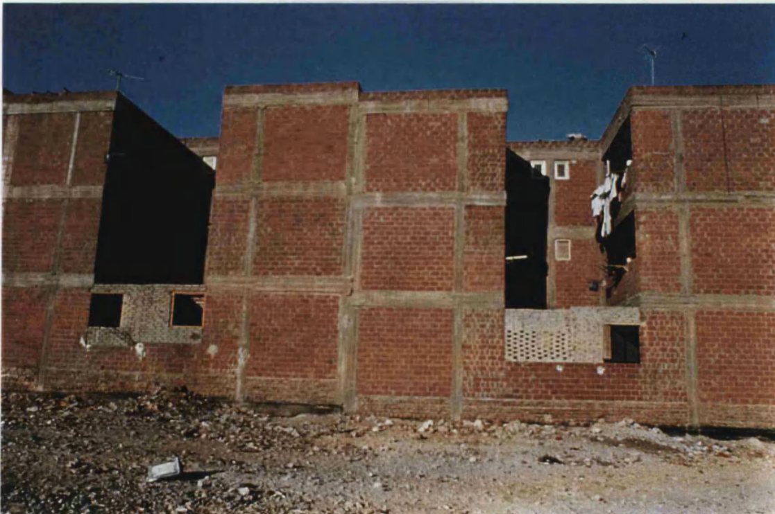
The second stage of appropriating extra space through the construction of outer walls - Neighbourhood 5 (1990)
