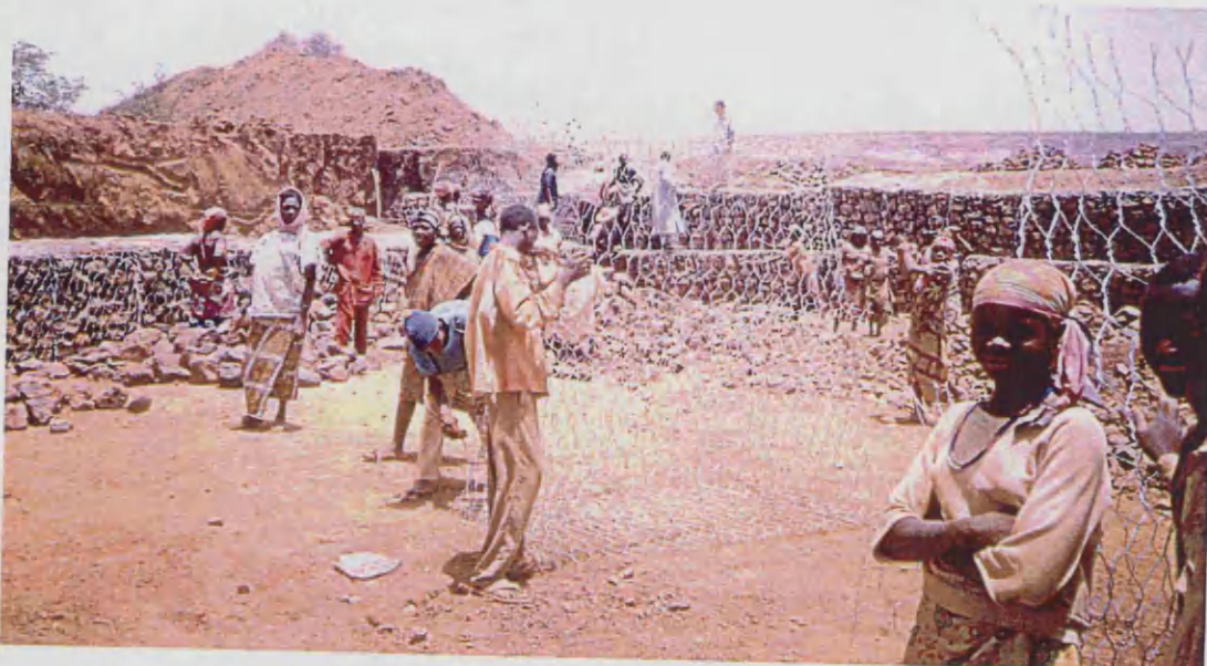
Picture 21 - Workers installing the gabions during the construction of a dike.
