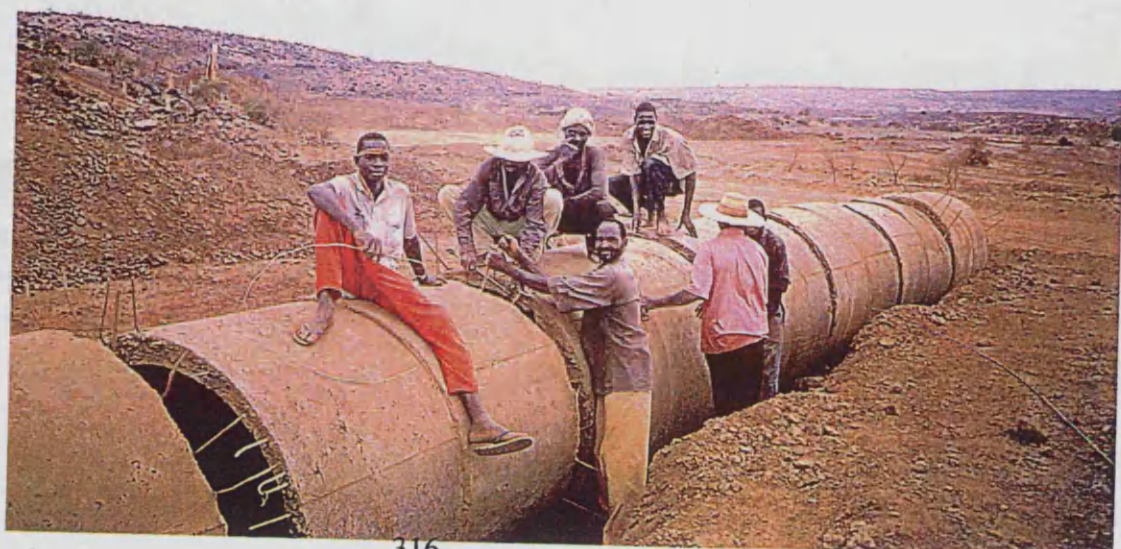
Picture 22 - Workers assembling the spillway of an earthfill dam.
