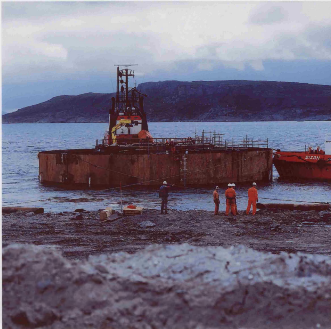
Deconstruction of the Brent Spar: A sliced segment of the storage tanks
