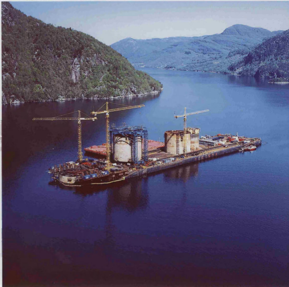
Deconstruction of the Brent Spar: Sliced parts of the storage tanks being transported ashore
