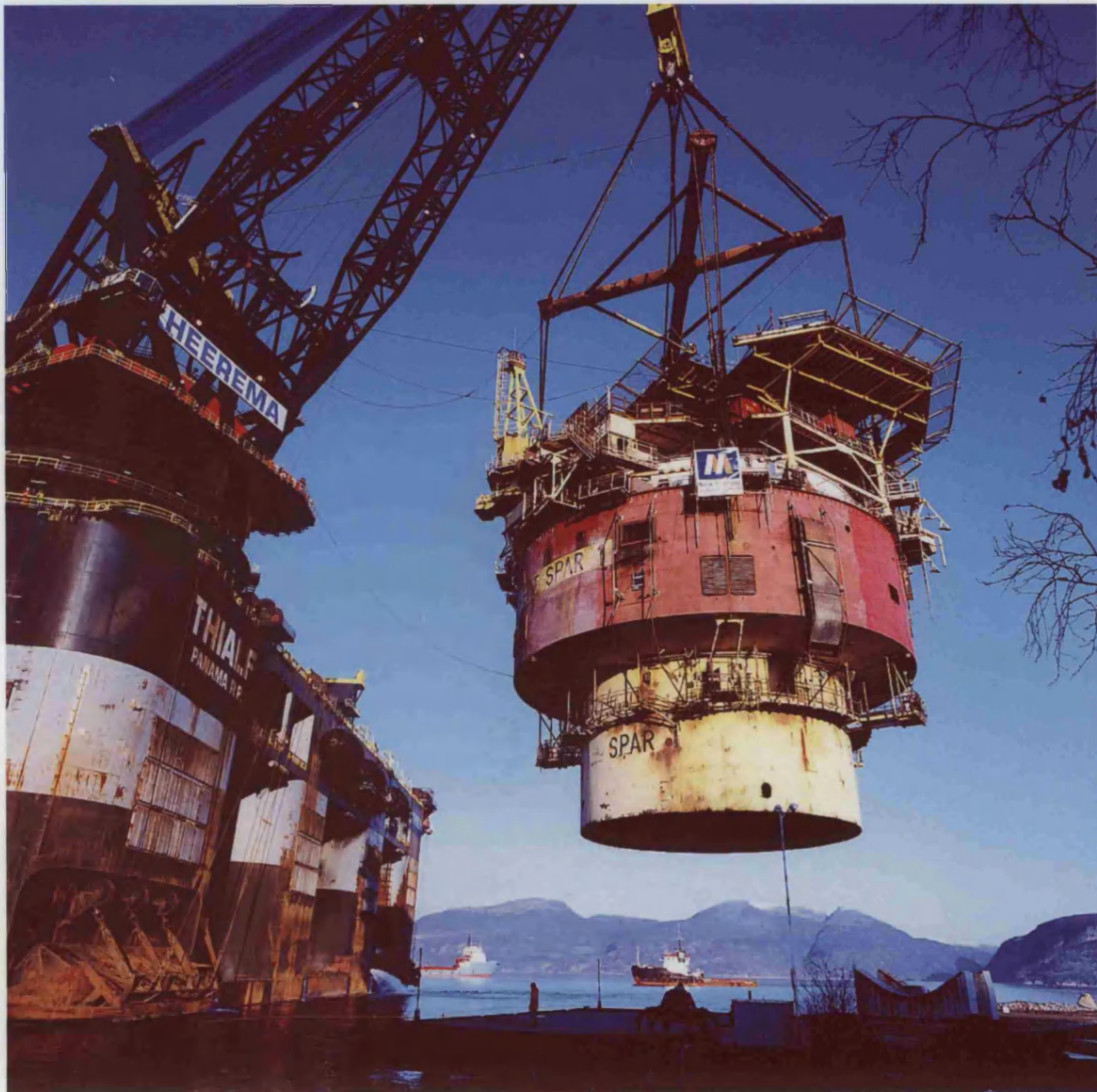
Deconstruction of the Brent Spar: Top part of the Spar separated from the storage tanks
