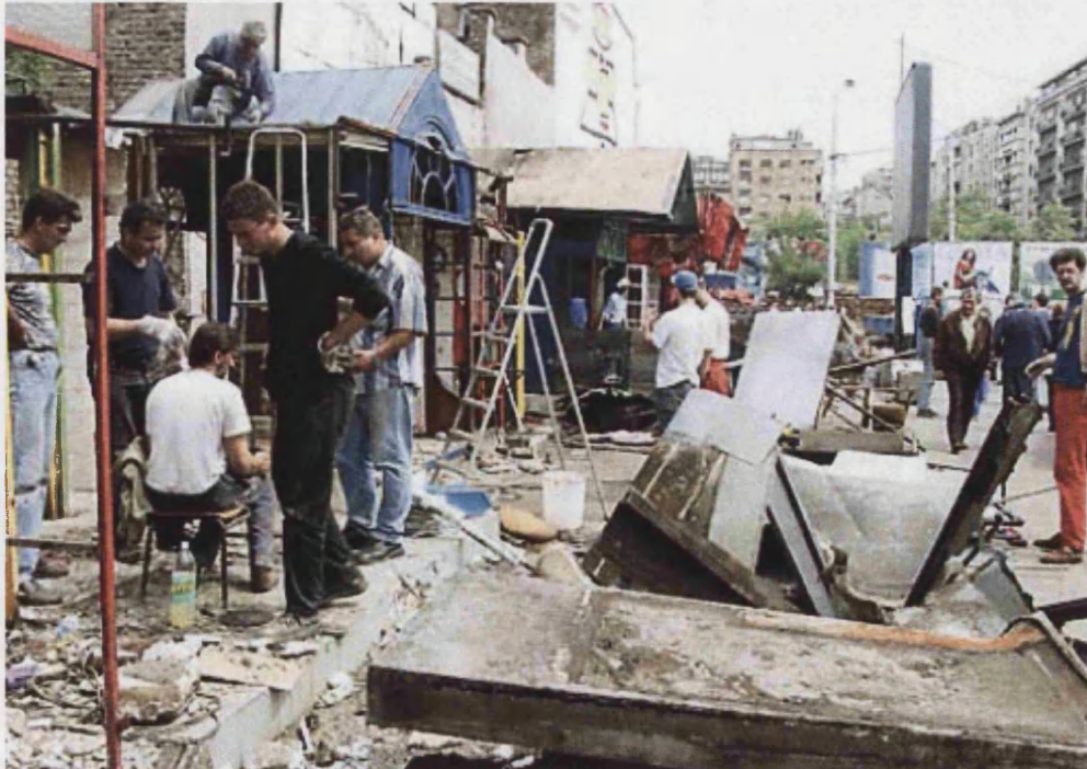
Picture 13: Demolition of numerous kiosks on pavements and central squares in 2002
