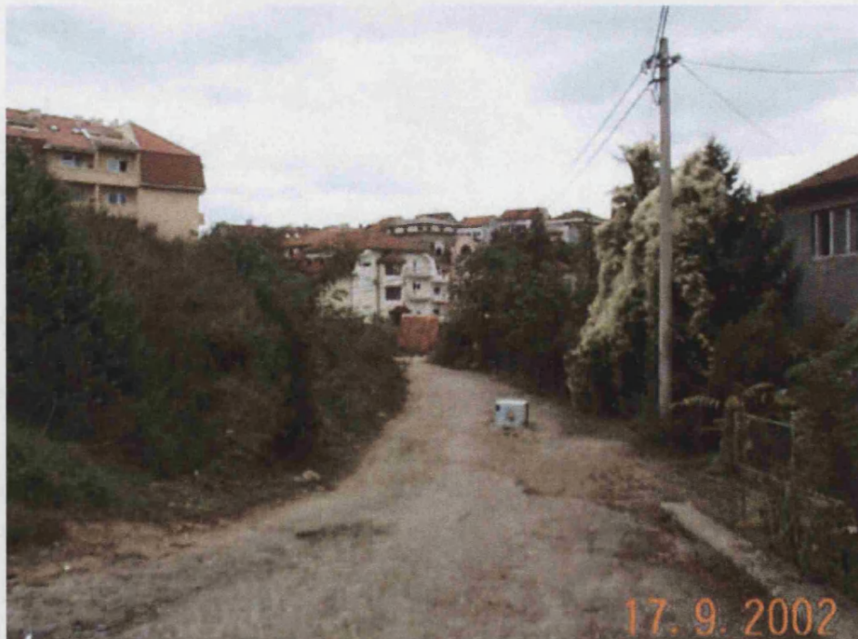
Picture 11: New residential area without streets and arranged public space
