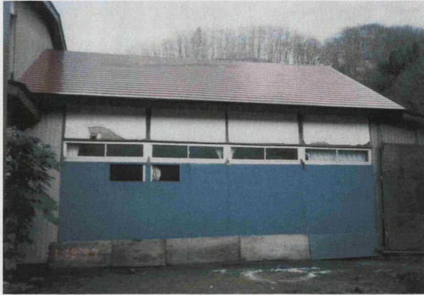
Figure 16. Windowpanes enclosed with wooden plates to protect them from the pressure of the snow
