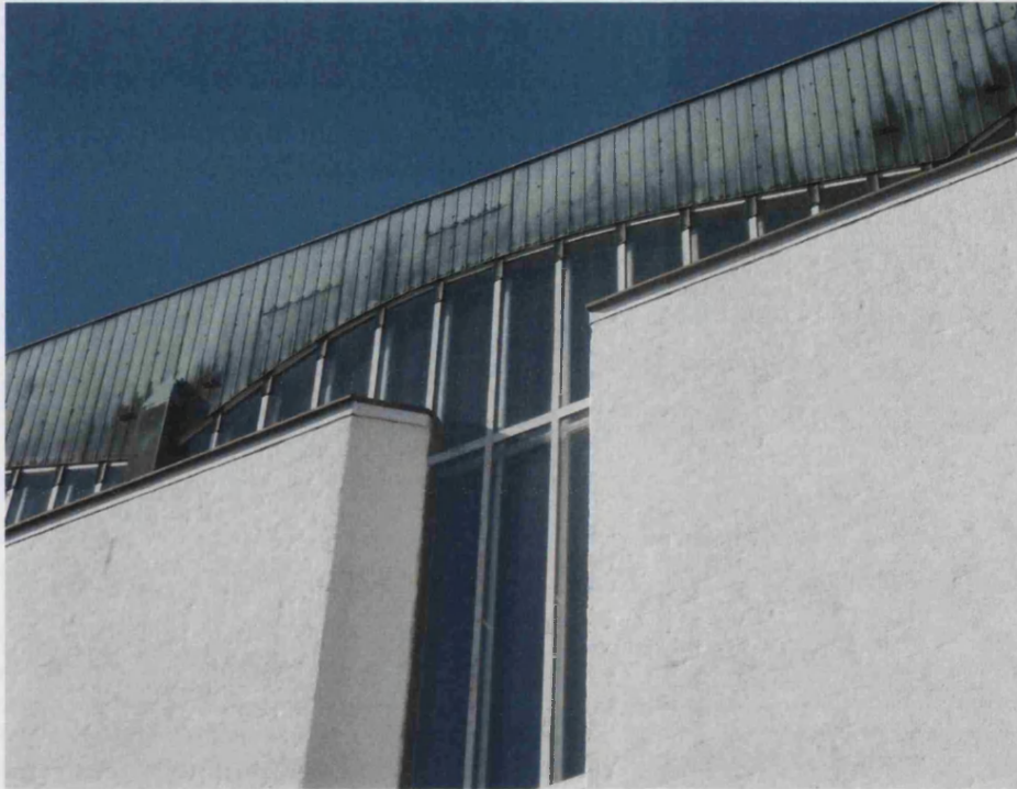
fig 5.23c Church thin-wash plastered brickwork, midday April 2005
