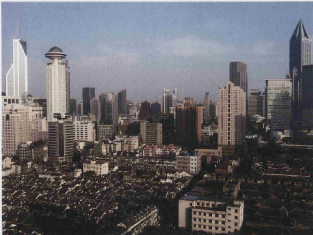
Figure 1.4: Low-rise 'lilong' housing in downtown Shanghai
