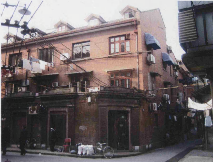
Figure 6.2: External view of rehabilitated lilong housing
