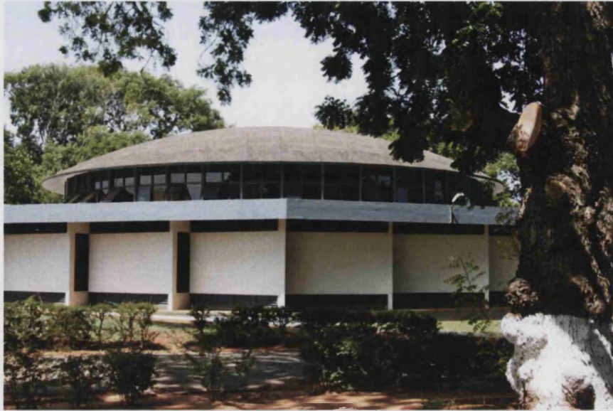
Figure 3.2. The main, dome-shaped building of the Ghana National Museum
