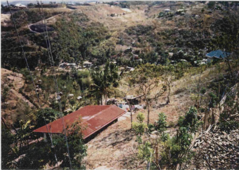
Plate 6.2 Mixed Housing Development in Buhisan
