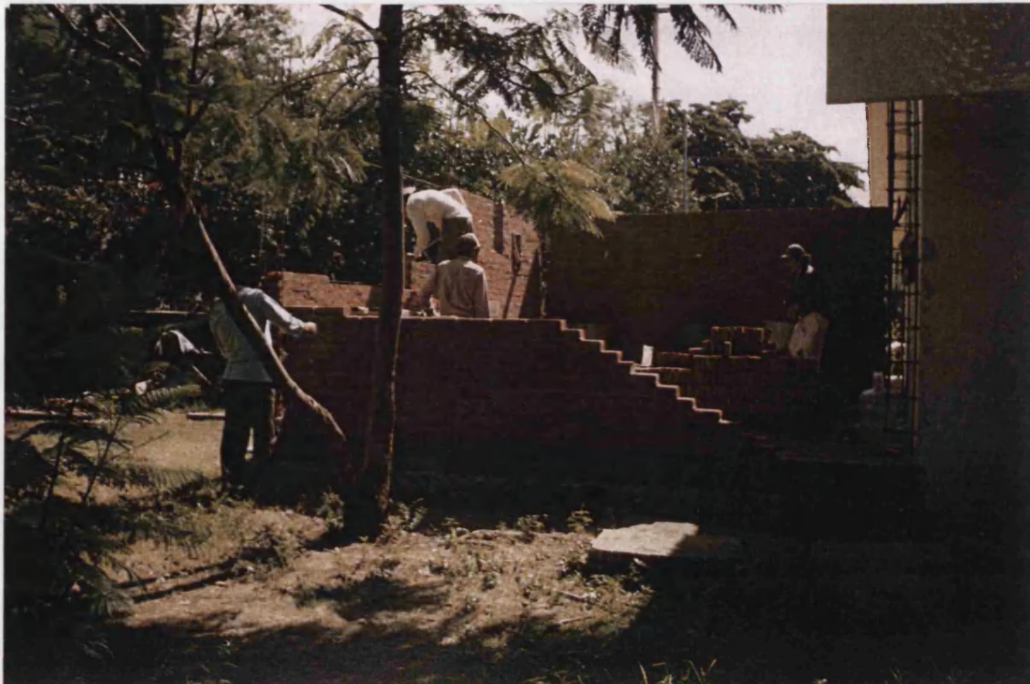
Photograph 2 Stage of the dental clinic construction when intervention began.
