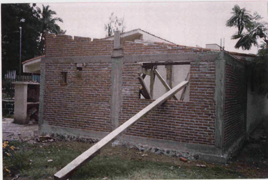
Photograph 6 The building ready for roof work
