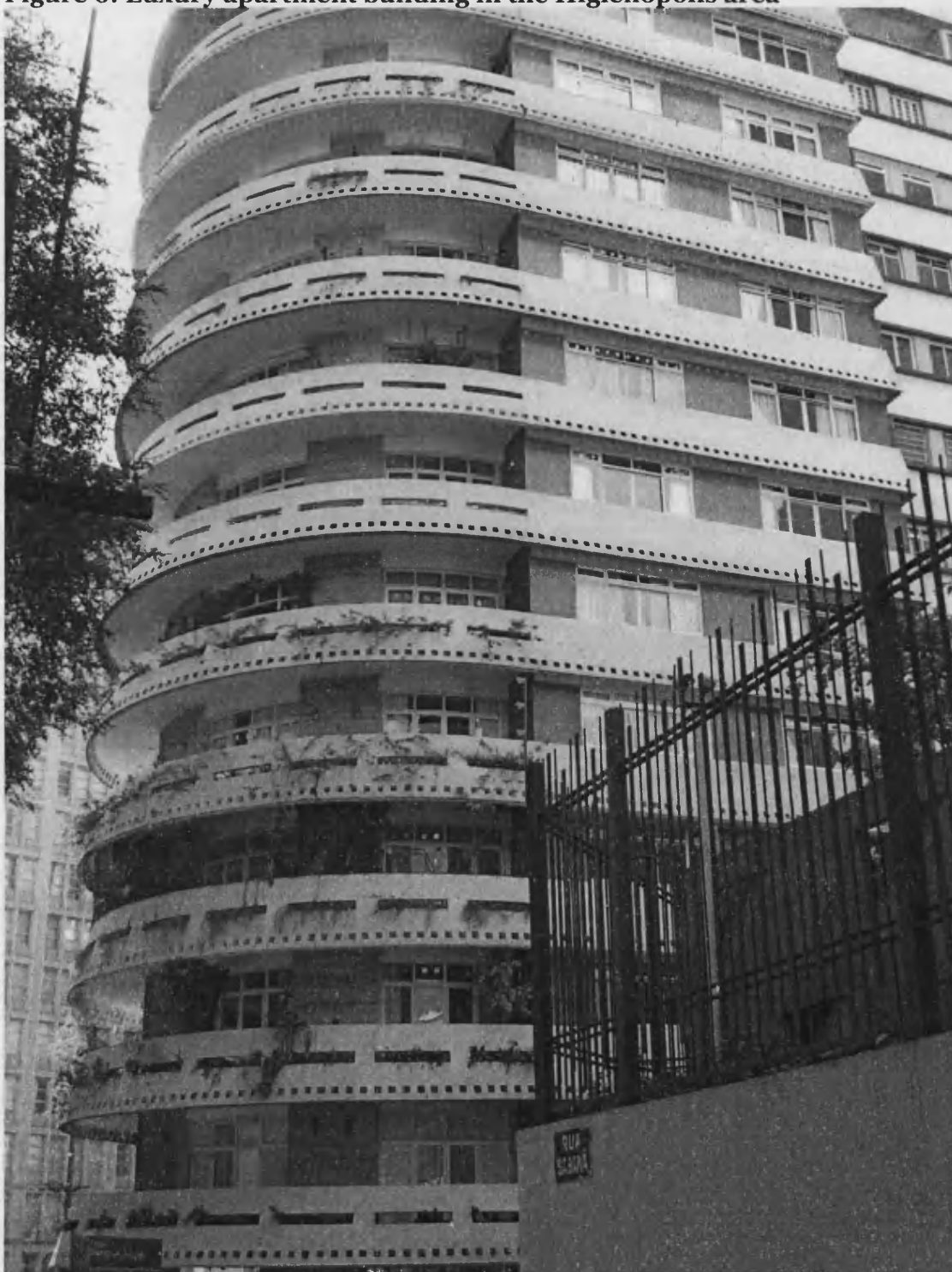
Figure 6: Luxury apartment building in the Higienópolis area
