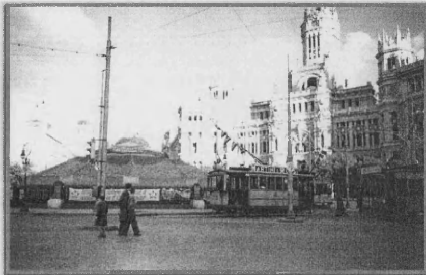
Fig. 6.8 Protective structure covering the fountain La Cibeles with the Palacio de Correos (the Postal Palace) in the background during the war (adapted from the web).
