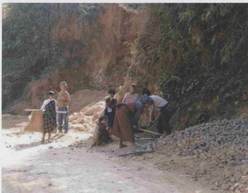
Picture 8: Households engaged in road construction in Nonglang Village (Fieldwork 2005)
