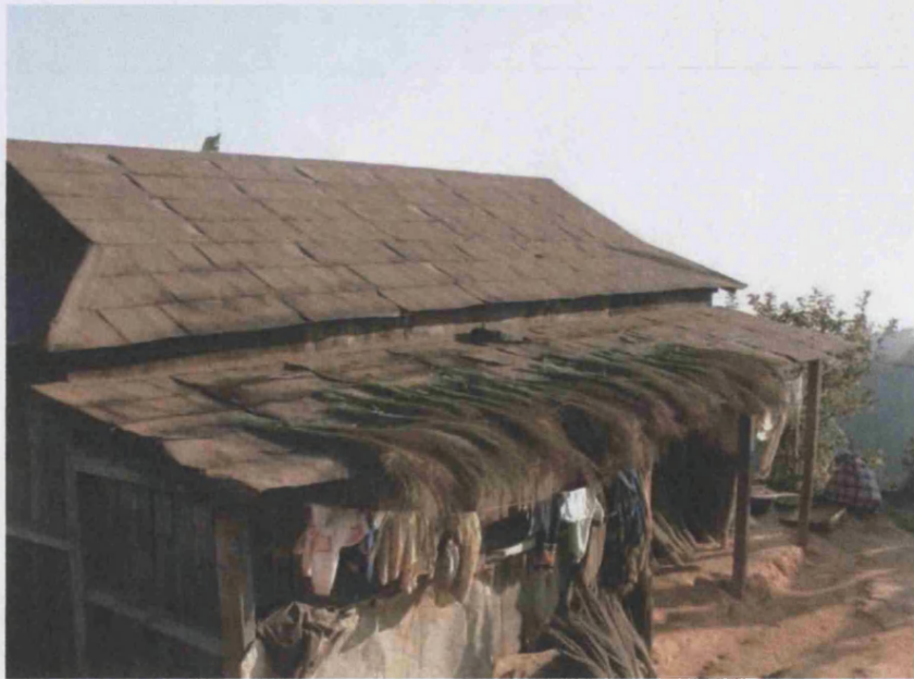
Picture 6: Drying of broom grass on rooftops in Nonglang Village (Fieldwork 2005)
