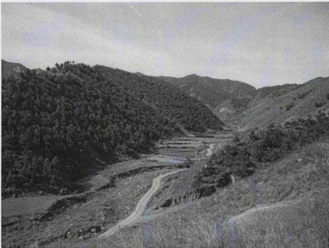
Picture 2.1 Xitai- before Sky's construction work in 2007
