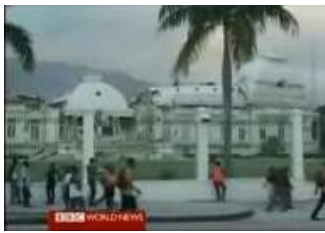
Figure 7-7: At the presidential palace, proof of the strength of this quake. It wasn't just flimsy buildings which collapsed. The central cathedral caught fire, it now lies in ruins.
