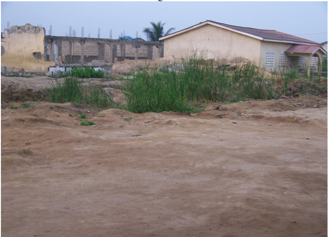
Figure A7: Abandoned Excavation for a Classroom Block, with an Additional Unfinished Classroom Block in the Background
