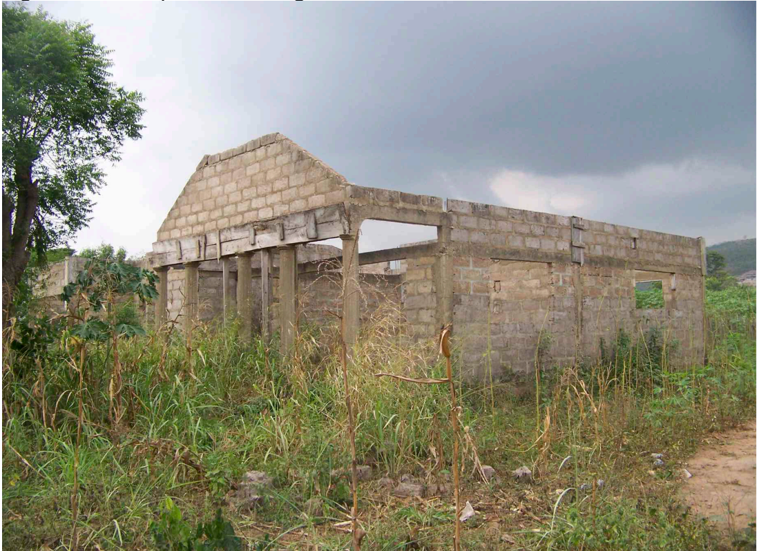
Figure A6: Incomplete Staff Bungalow
