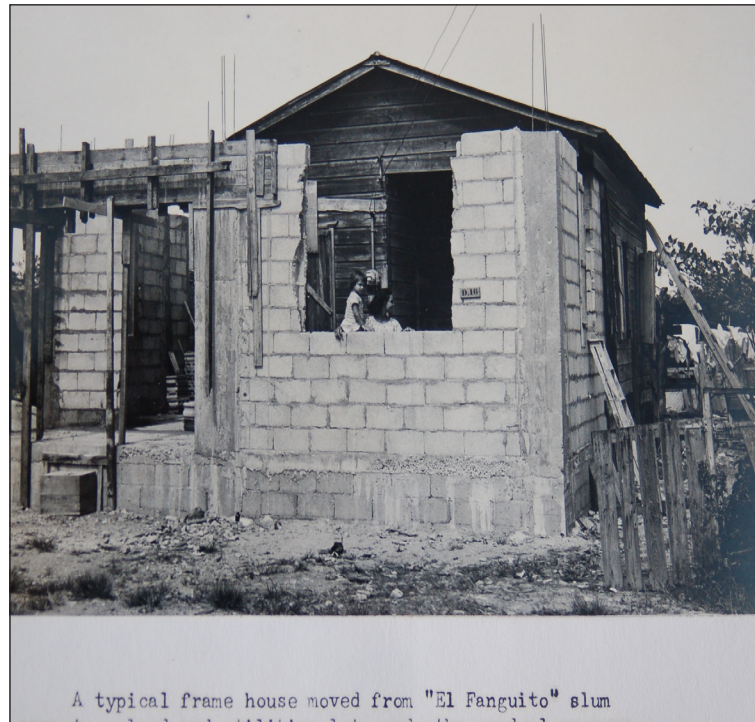
Figure 4.4. 'A typical frame house'. Source: Puerto Rico Housing Authority Memo. Dec.16, 1955. CIP/ AGPR/ ICP
