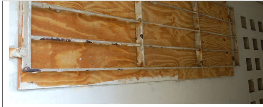
Figure 5.14. The effects of vandalism: this boarded window is one of the precarious effects of vandalism, with a mere wooden plank separating the space of the abandoned apartments and the hallways. This had become a common feature of many of the building's windows and a symbol of residents' new sense of insecurity. The boards were pointed out frequently to me as evidence of how bad things were. Source: Author.
