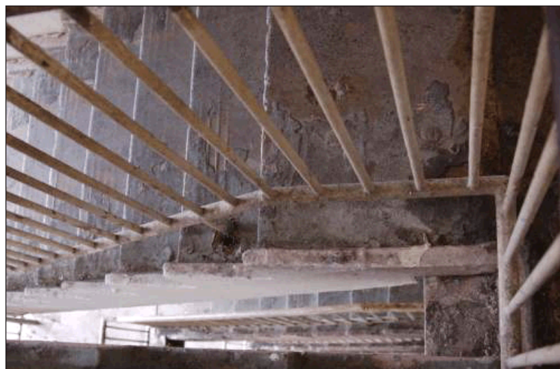
Figure 6.18. Image of rusty stairs in Gladiolas, Tower B. 2007. Source: Author.
