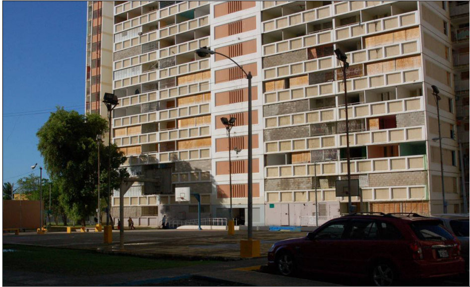
Figure 1.8. Entrance. Gladiolas II, courtyard, parking lot and Tower 301. Source: Author.
