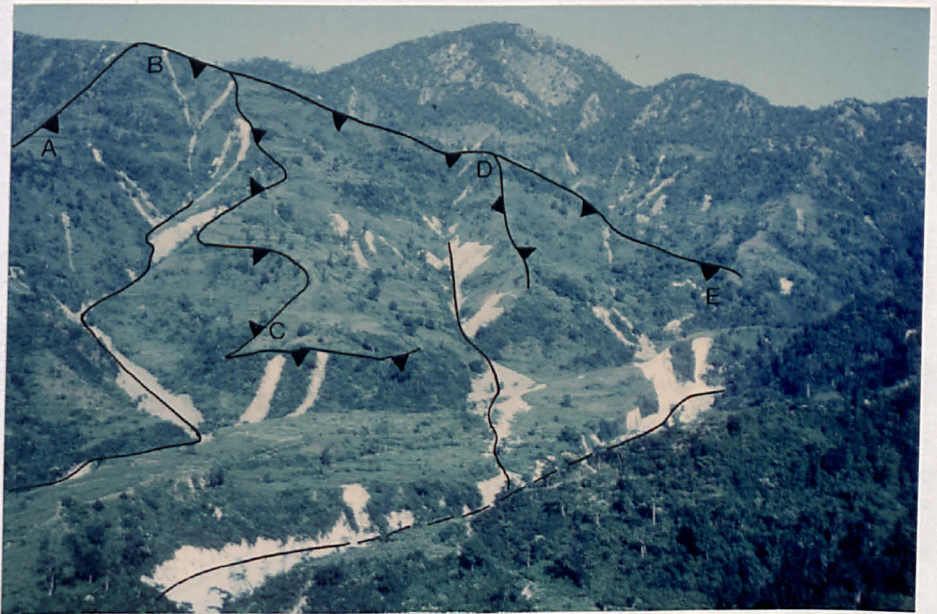
PLATE 4.5 Slopes Crossed by the COALMA Line on the Western Flanks of the Sardu Khola:Post-1984 Storm.
