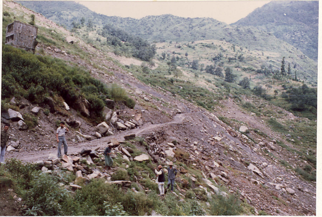
PLATE 2.7 Rotational Slope Failure Causing Gradual Slope Displacement Along the Kathmandu-Kodari Road.
