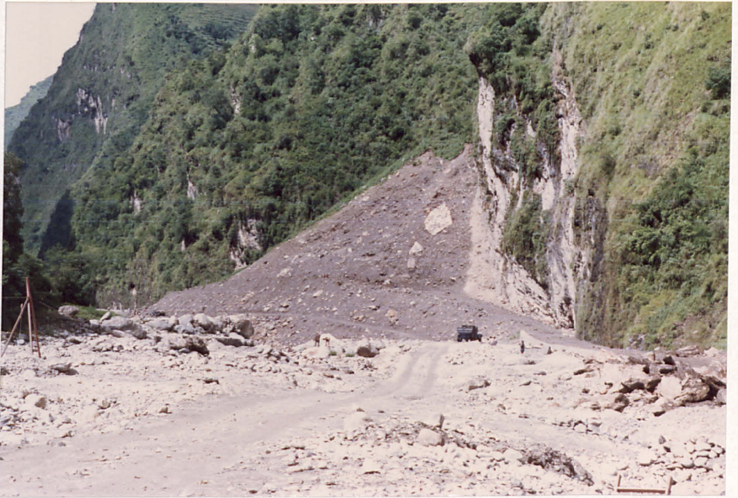
PLATE 2.5 Debris from Large Translational Failure Engulfing Part of the Kathmandu-Kodari Road.
