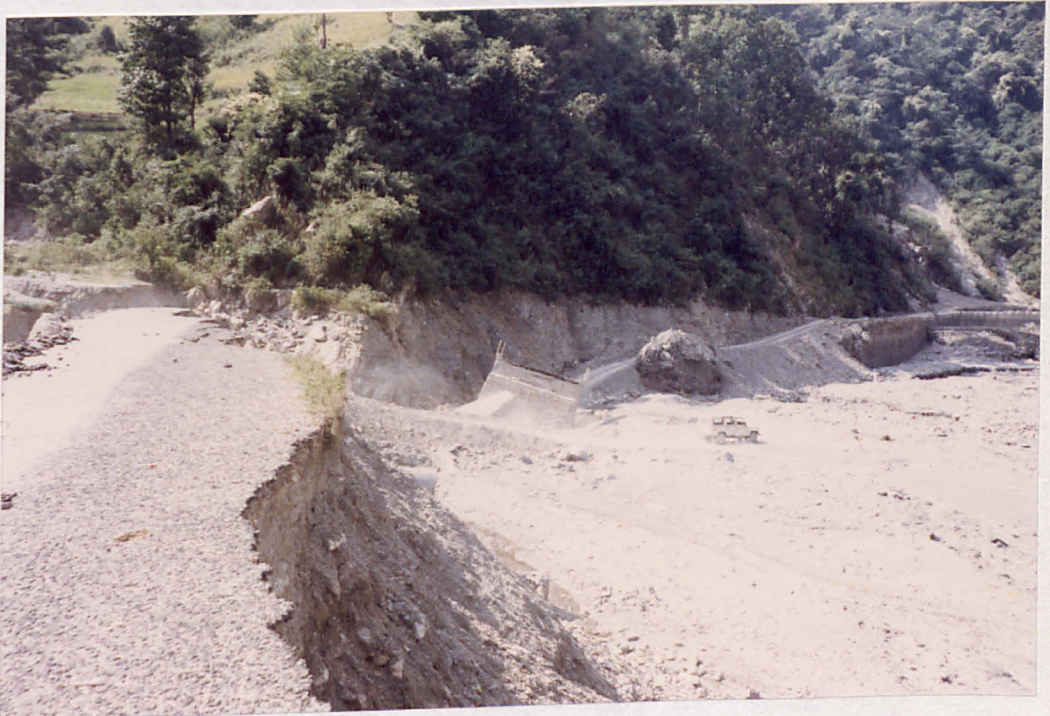
PLATE A.6 Road Loss at Km 28.100 on the Leoti Khola Floodplain.
