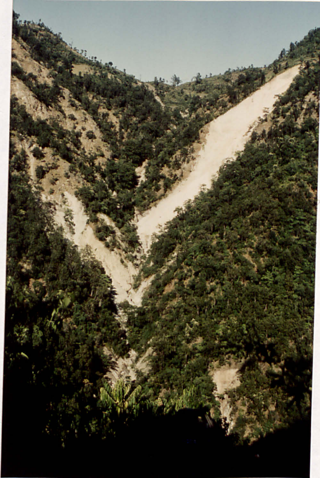
PLATE 4.3 Rock Slide in Quartzite Along the COALMA Line, Initiated During the 1983 Monsoon.
