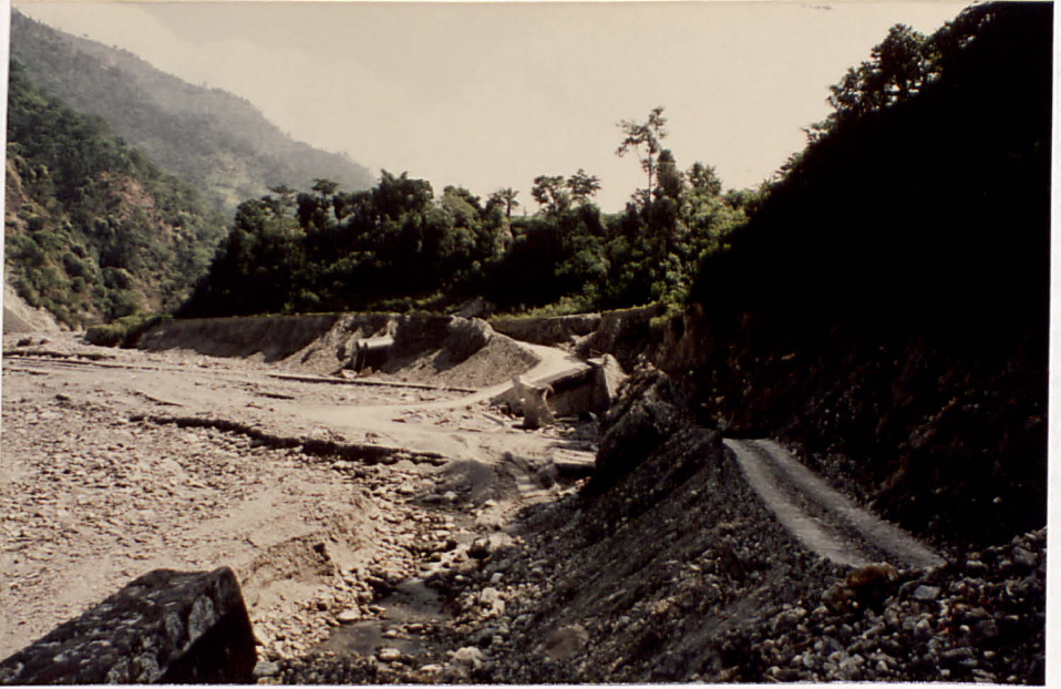
PLATE 2.9 Extensive Damage to the Dharan-Dhankuta Road Caused by Flooding in the Leoti Khola in 1984.
