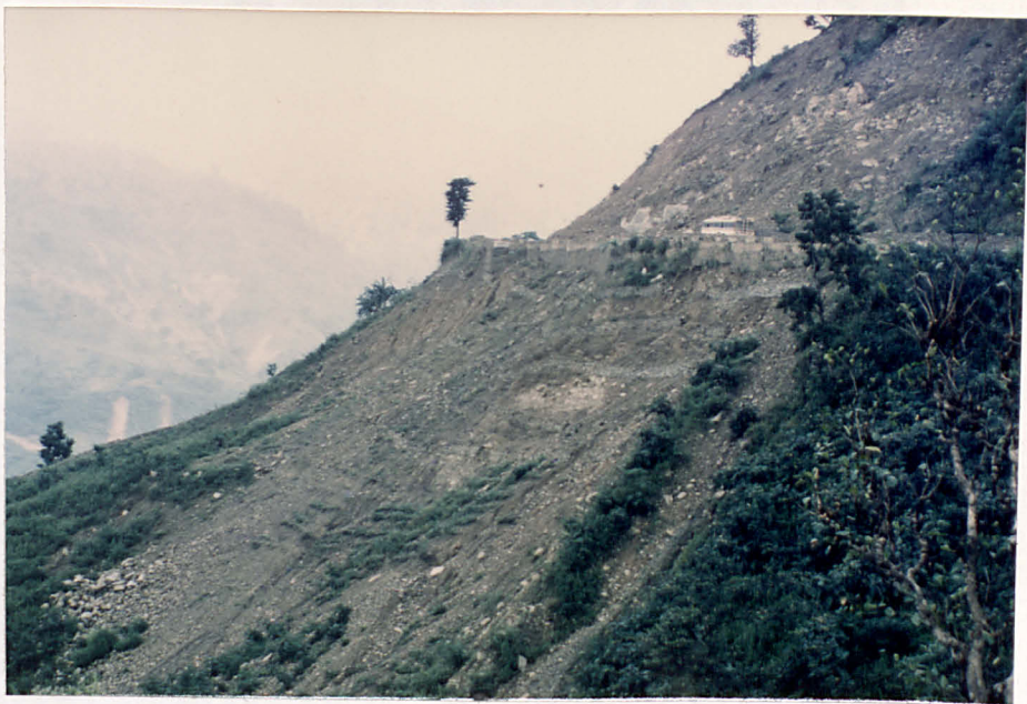
PLATE 2.15 Deep-Seated Rotational Failure at Km 4.100 on the Dharan-Dhankuta Road in September 1983.
