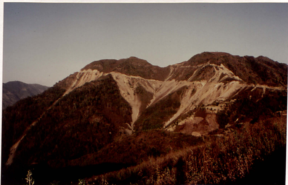
PLATE 6.4 Extent of Bare Ground Caused by Side Casting Along the Bhedetar-Rajarani Road in 1983.
