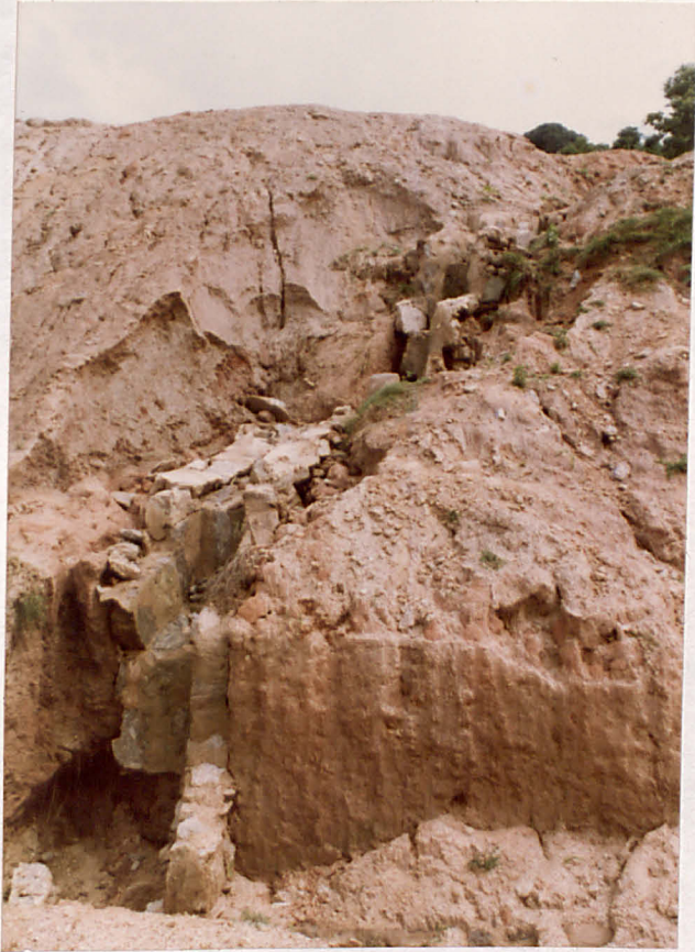
PLATE A.7 Undermining of Area Drainage by Erosion on the Gneiss Slopes Below Dhankuta.
