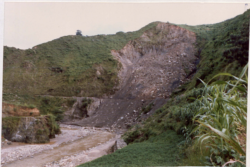
PLATE 2.3 Renewed Instability on Meander Bend Along the Kathmandu-Kodari Road, Reactivated by Road Excavation.
