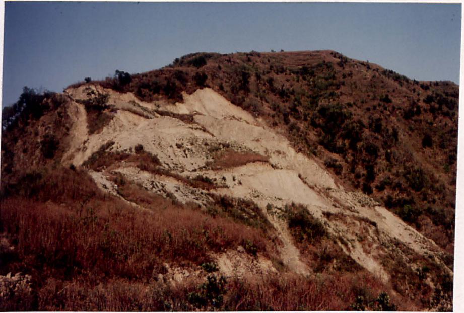
PLATE 6.6 The Obliteration of a Hairpin Stack Along the Original Alignment for the Bhedetar-Rajarani Road Following Extensive Spoil Tipping.
