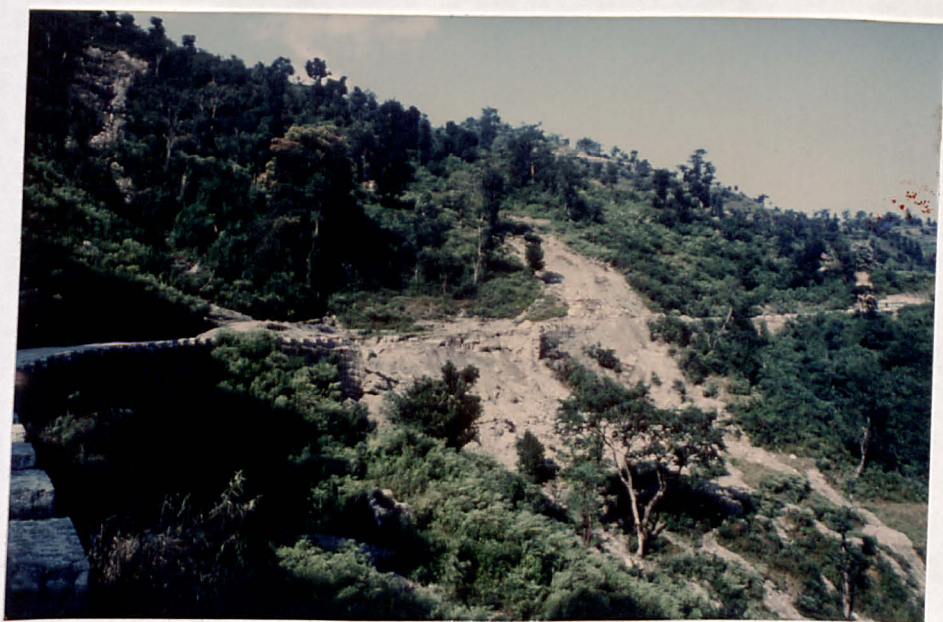
PLATE 2.16 Road Loss by Debris Flow at Km 23.400 on the Dharan-Dhankuta Road.
