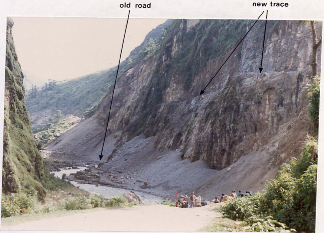
PLATE 2.17 Location of the Kathmandu- Kodari Road in the Engorged Bhote Kosi Valley. (Following Removal of the Road by Flooding, the Alignment has been Relocated Further up the Gorge Flank in Full Cut).
