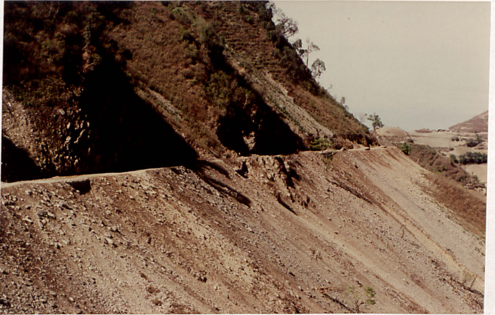
PLATE 6.3 The Bhedetar-Rajarani Road Along the Study Section, Showing the Full Cut Excavation and Side Casting of Spoil.
