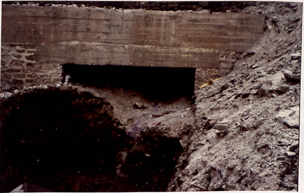
PLATE 2.10 Culvert Blockage Along the Dharan-Dhankuta Road.
