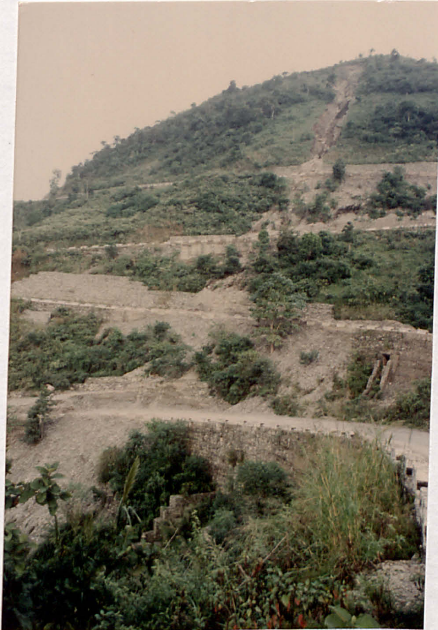
PLATE A.2 Debris Flow Deposits on the Kumlintar Hairpins.
