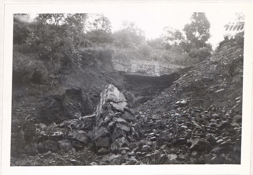
PLATE A.4 Erosion Below Side Drain Exit on the Descent to the Leoti Khola Floodplain.
