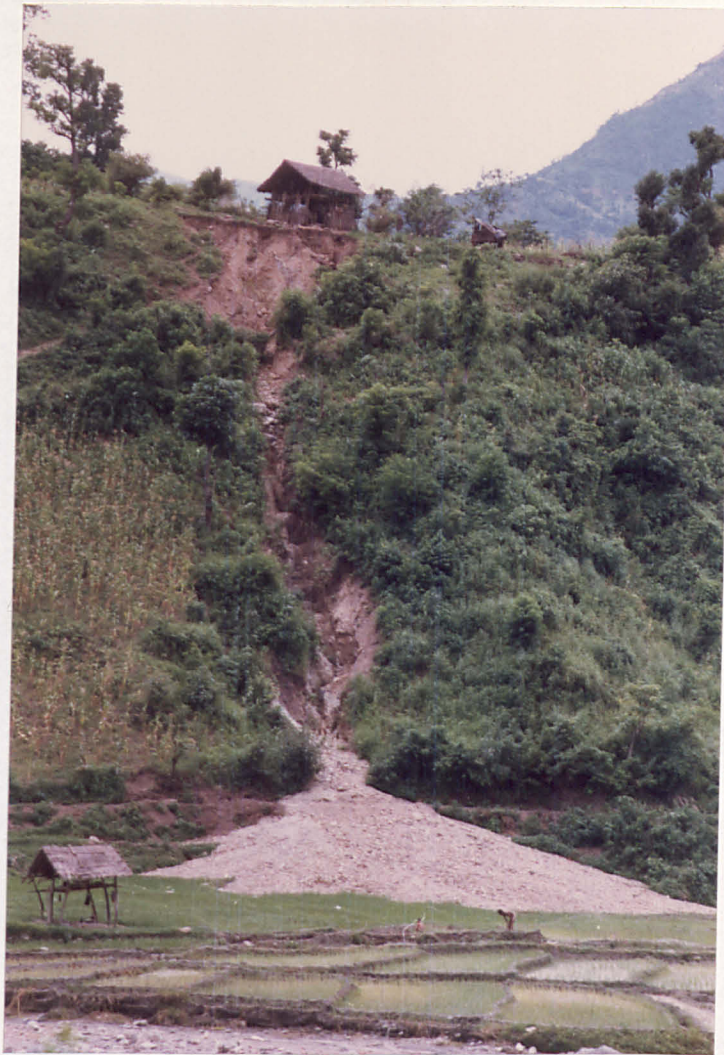
PLATE 2.2 Debris Fan Below Eroding Gully in East Nepal.
