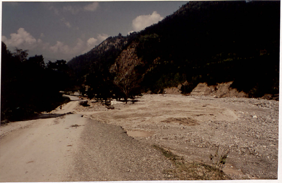
PLATE A.5 Partial Burial by Sediment of the Road Camp at Phalametar, on the Leoti Khola Floodplain.
