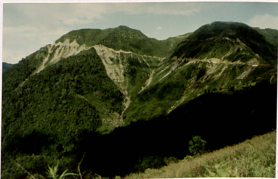
PLATE 6.5 Extent of Bare Ground Caused by Side Casting Along the Bhedetar-Rajarani Road in 1984.
