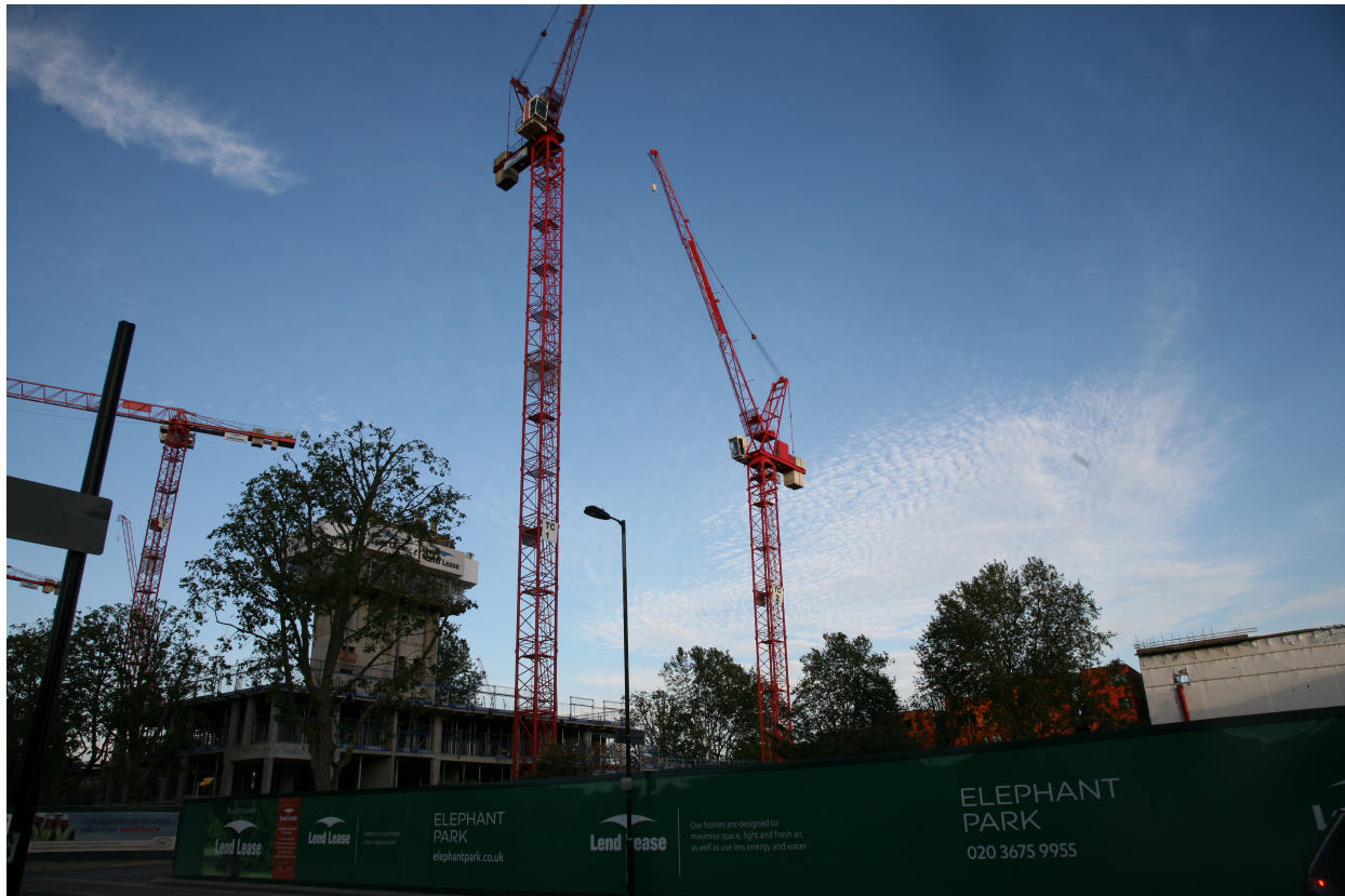
Figure 36: Construction site, Elephant Park
