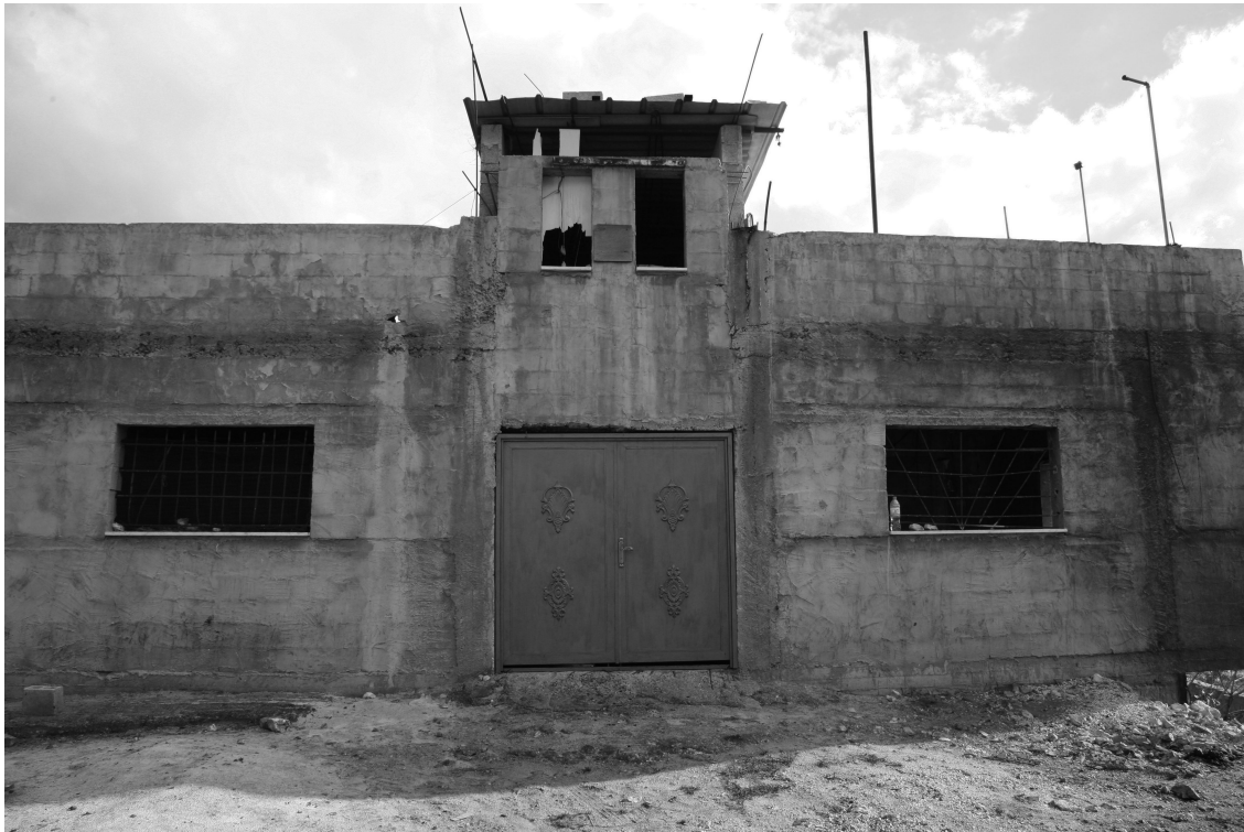
Figure 19: Home in Area C showing firebomb damage. The home is still lived in.
