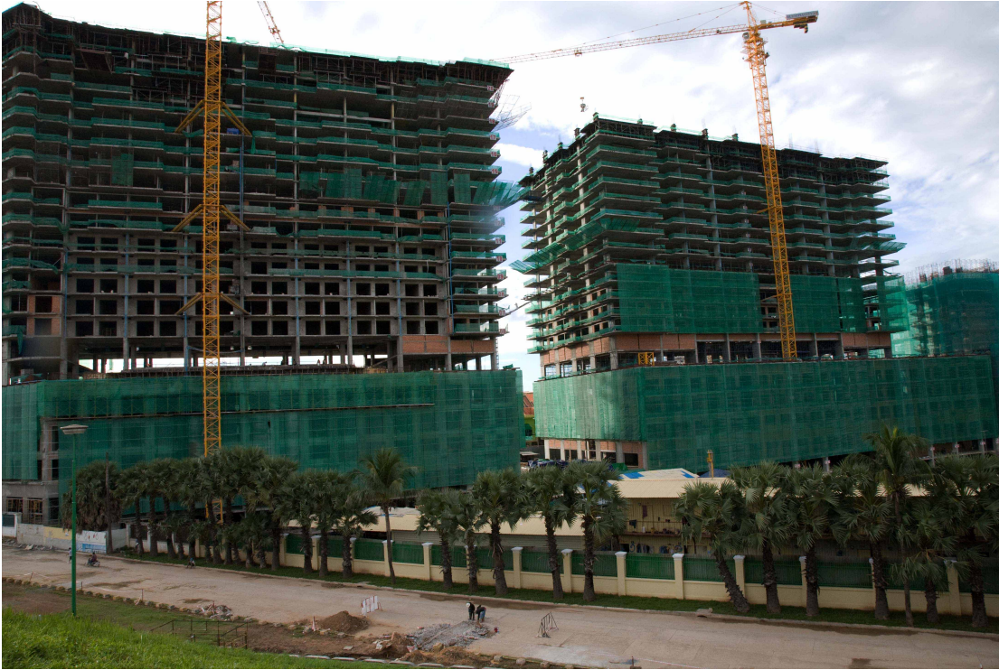
Figure 15: Construction in Phnom Penh
