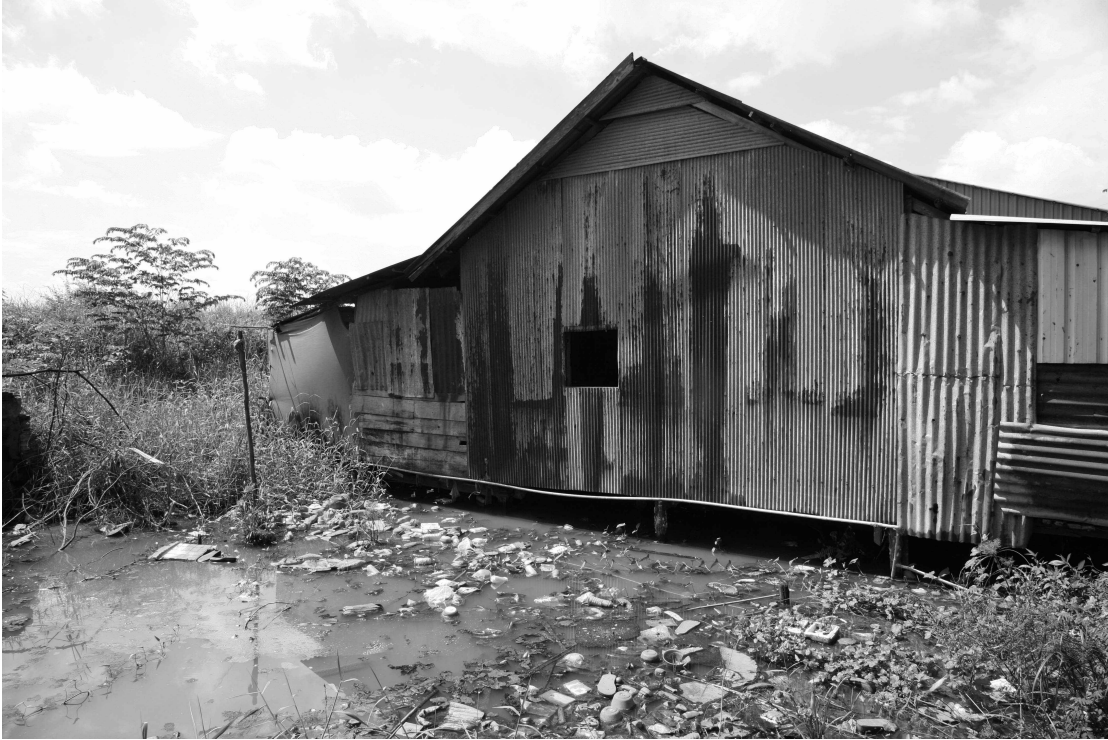
Figure 8: Flooding and subsidence
