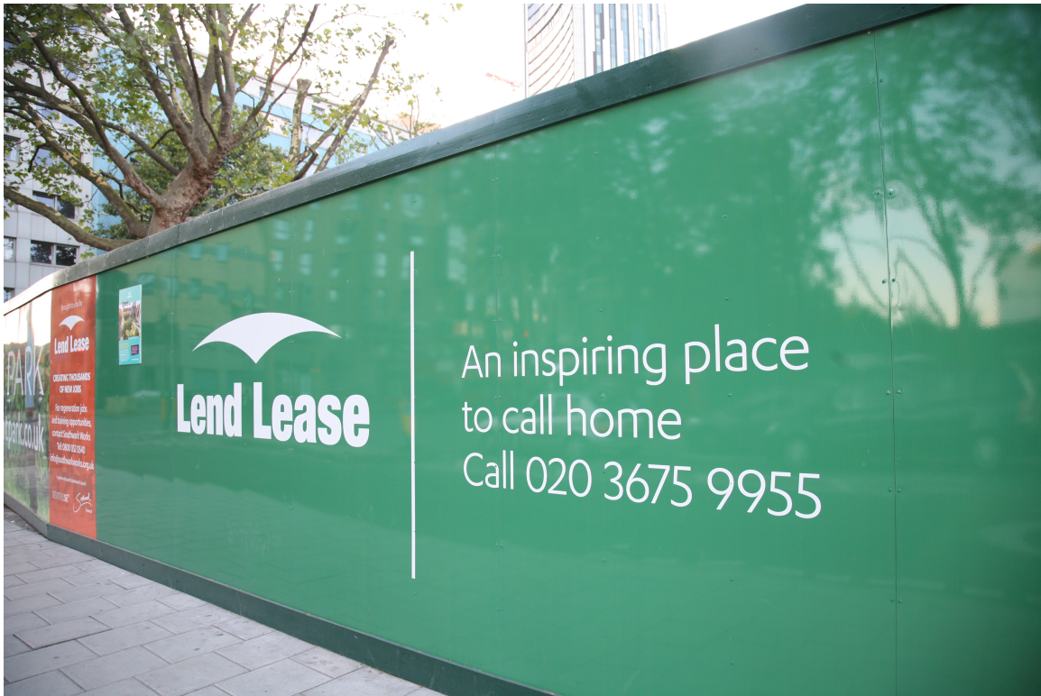
Figure 35: Construction hoarding at Elephant Park
