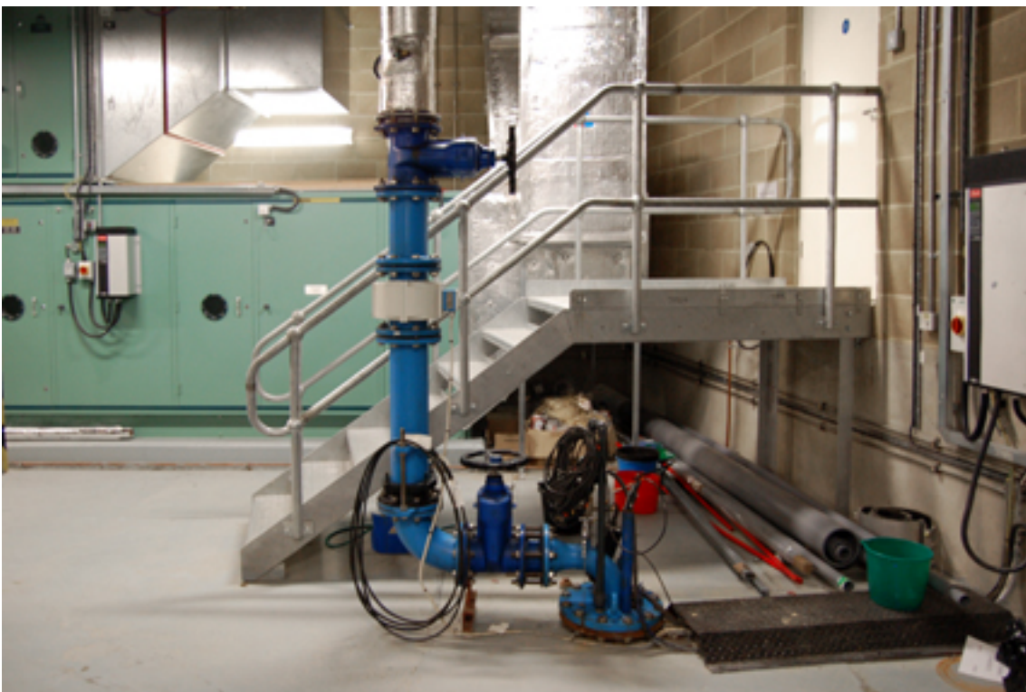
Figure 7.4 City Hall's main plant room with the arrival point of the borehole extraction pipe in the front (Photograph: Author, 2011)
