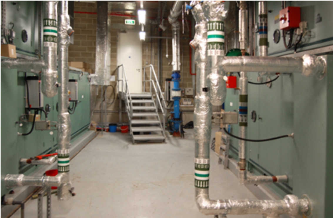
Figure 7.3 City Hall's main plant room with air handling units left and right (Photograph: Author, 2011)
