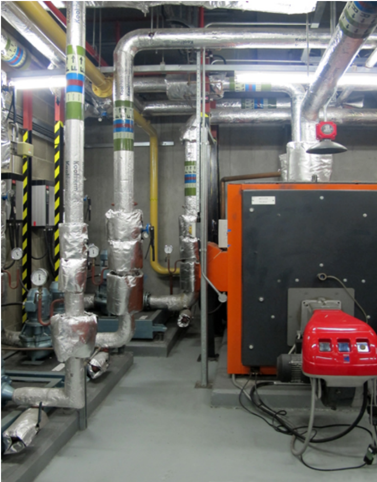
Figure 7.5 City Hall's boiler plant room in the basement (Photograph: Author, 2011)
