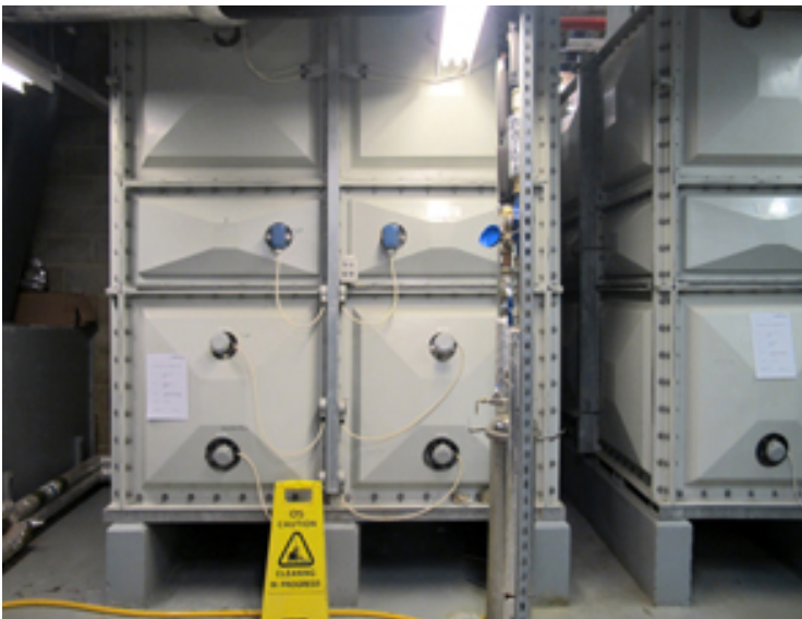
Figure 7.6 City Hall plant room in the basement with grey water tanks (Photograph: Author, 2011)
