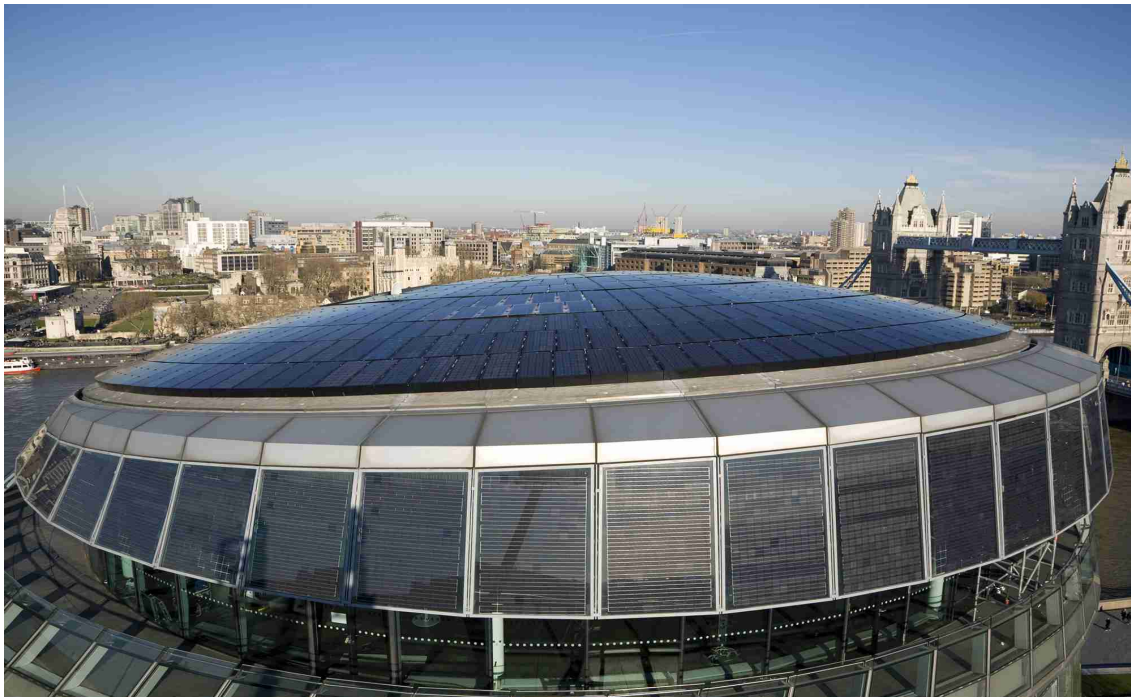
Figure 7.7 Photovoltaic modules on the roof and eyelash of City Hall (Photograph: Sunny Portal, 2012)
