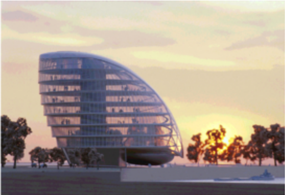
Figure 6.7 Planning Application scheme (Photograph: Richard Davies, 2004)
