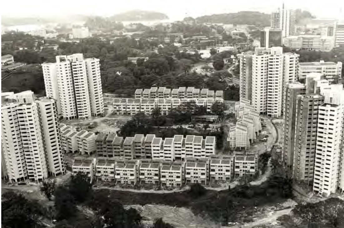
Figure 7-10 A panoramic view of Gillman Heights before its completion in January 1984
