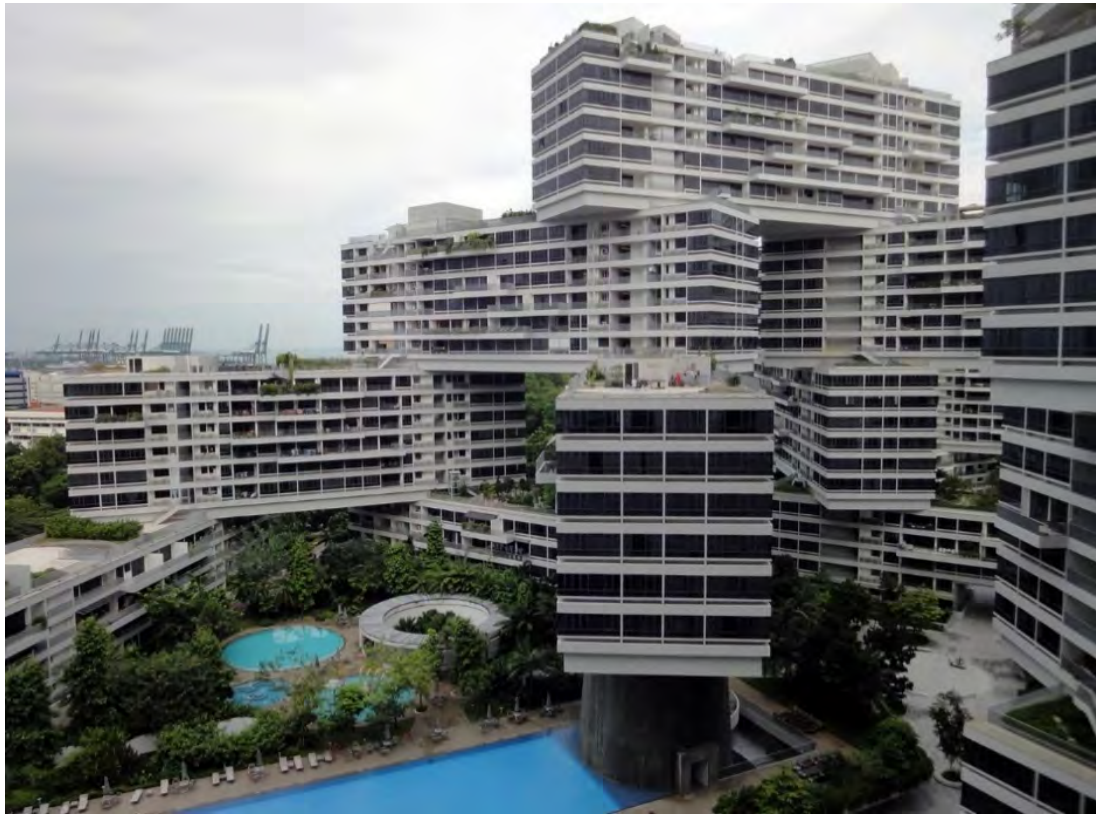
Figure 7-9 Overview of Interlace condominium
