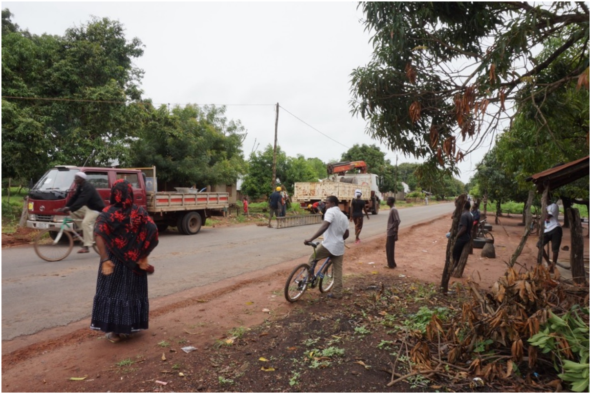
FIGURE 8 CONSTRUCTION OF THE MAIN GRID IN BAMBADINCA
