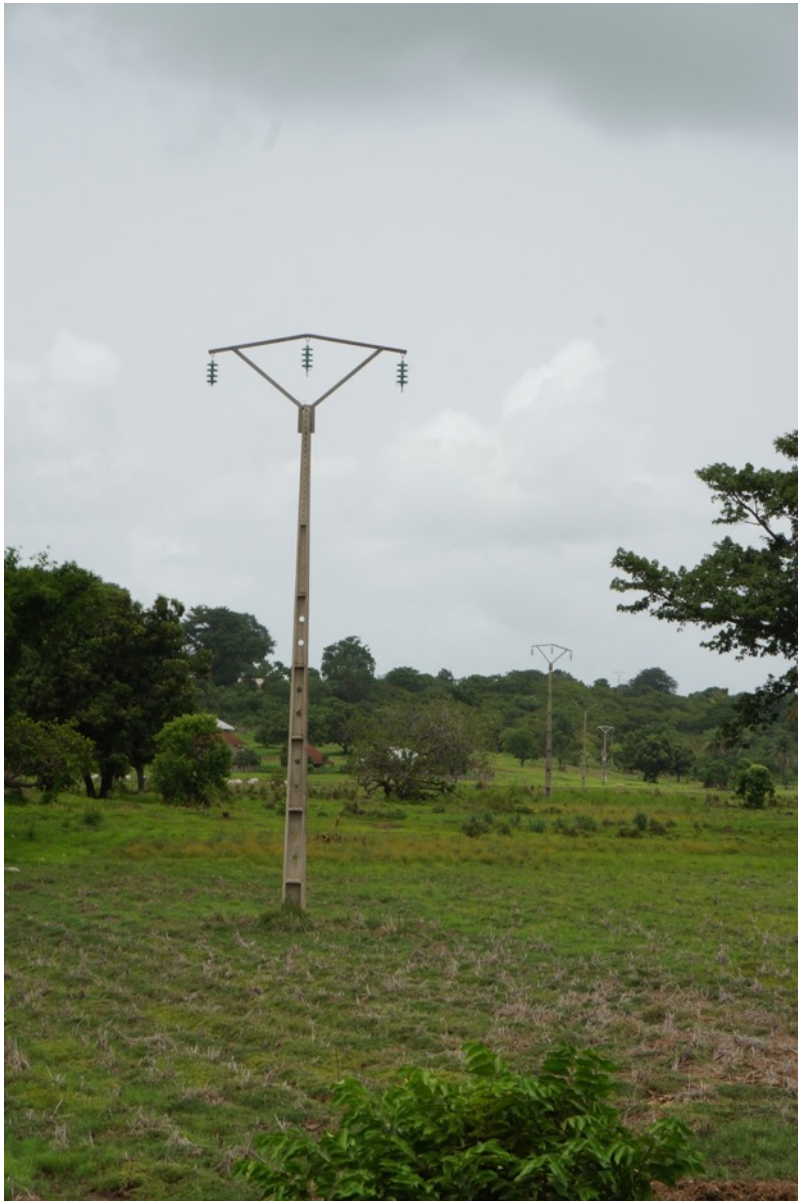
FIGURE 6 ABANDONED INFRASTRUCTURE IN BAMBADINCA THAT WAS LATTER INCORPORATED TO THE MAIN GRID
