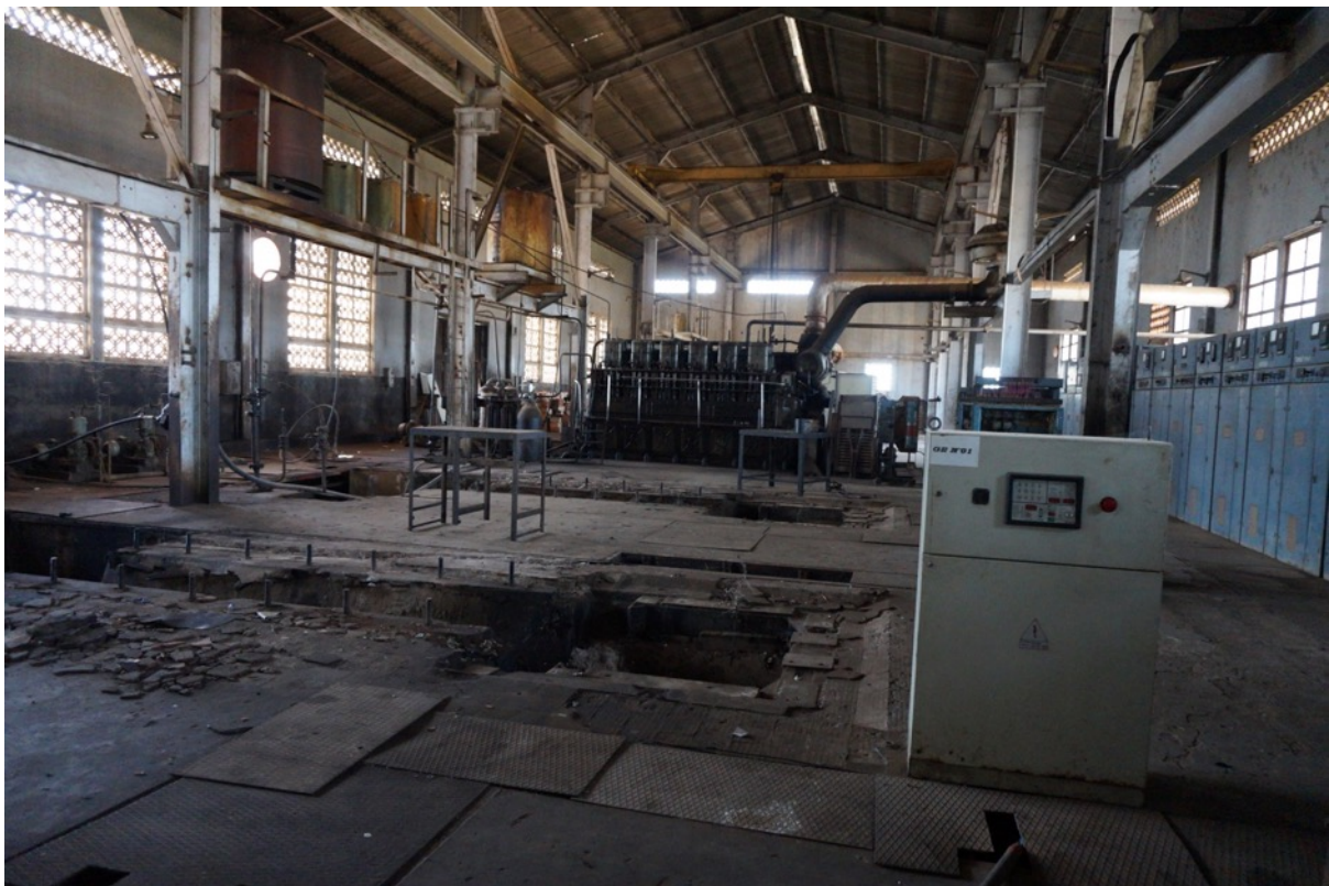
FIGURE 1 THE BAFATÁ CITY POWER PLANT THAT USED TO ELECTRIFY THE WHOLE REGION NOW OPERATES WITHIN THE LIMITS OF BAFATÁ CITY
