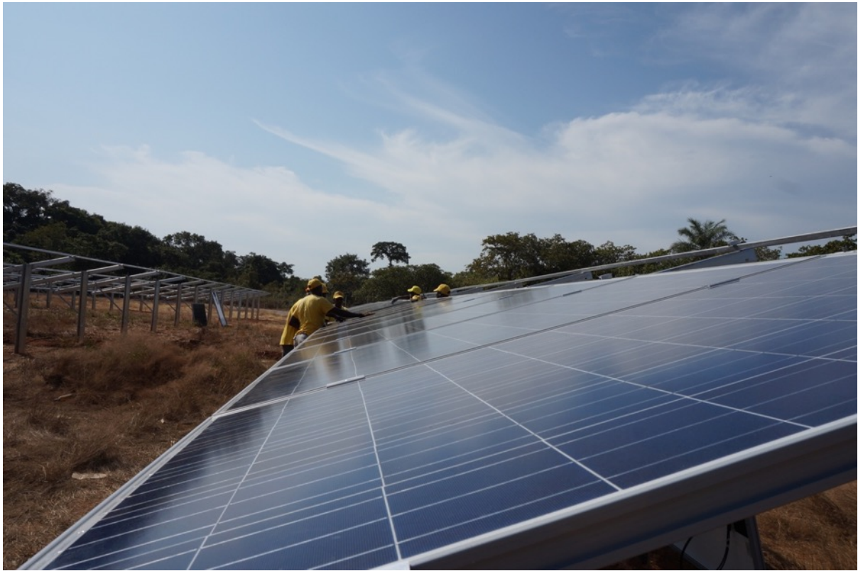
FIGURE 7 INSTALLATION OF THE SOLAR PANELS IN THE MINI-GRID STATION IN BAMBADINCA
