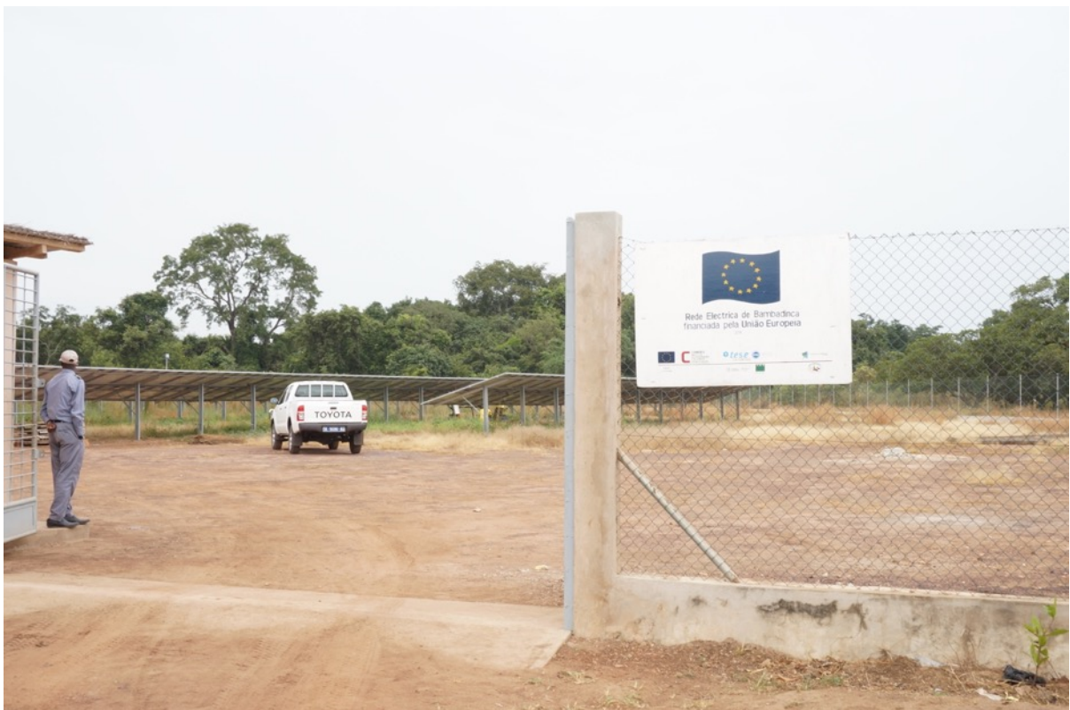
FIGURE 11 ENTRANCE OF THE MINI-GRID STATION IN BAMBADINCA
