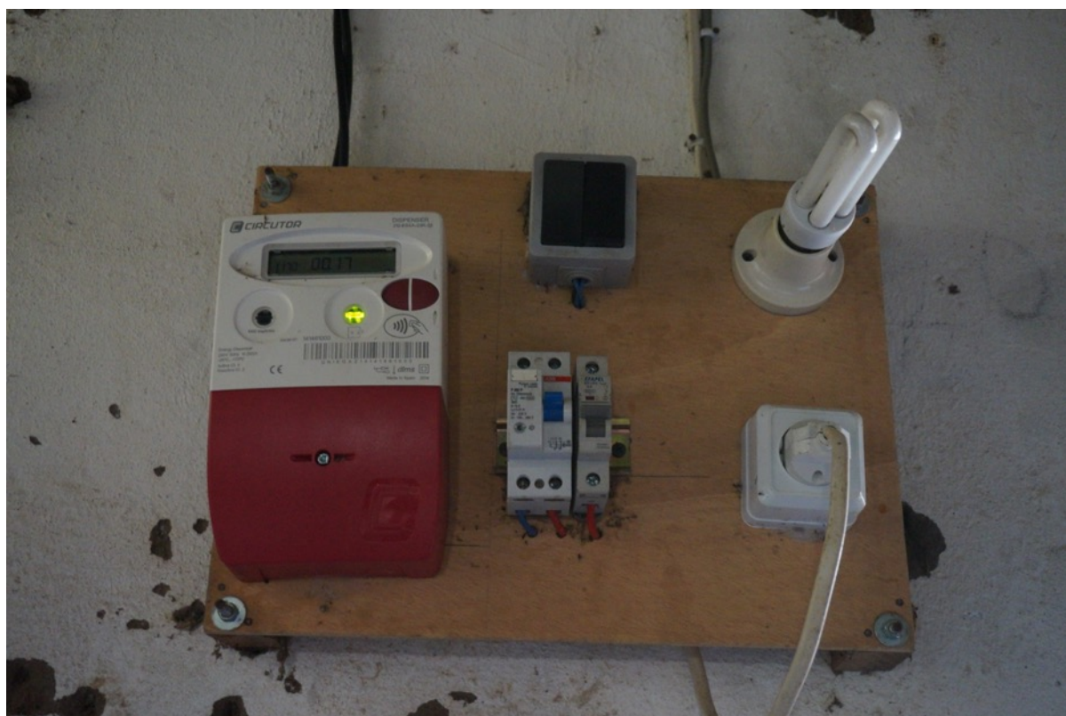
FIGURE 12 METER INSTALLED WITHIN THE HOUSEHOLD OF A CLIENT OF THE SERVICE IN BAMBADINCA. THE GREEN LIGHT INDICATES THAT THE CHEAPEST TARIFF IS BEING CHARGED
