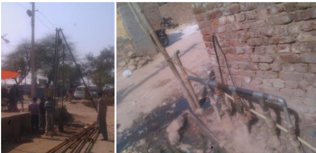
'Captured' tubewells, Sangam Vihar. The well on the right has pipes for four lanes and a personal connection for a local party worker's house
