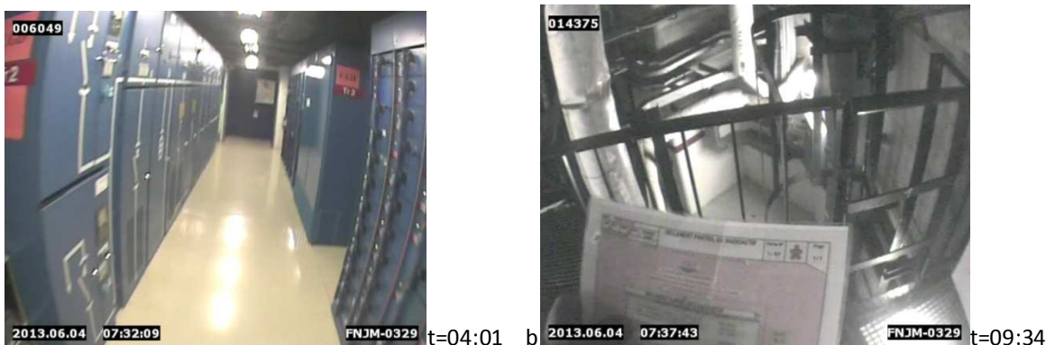
Fig. 34 a & b: Field worker performing isolation of steam generator #1 due to high level of radioactivity inside. Picture extracted from one of the subjective videos; in a) crossing a electric cells room, b) reading the MO and wondering whether or not he must descend the caged ladder in front of him.
