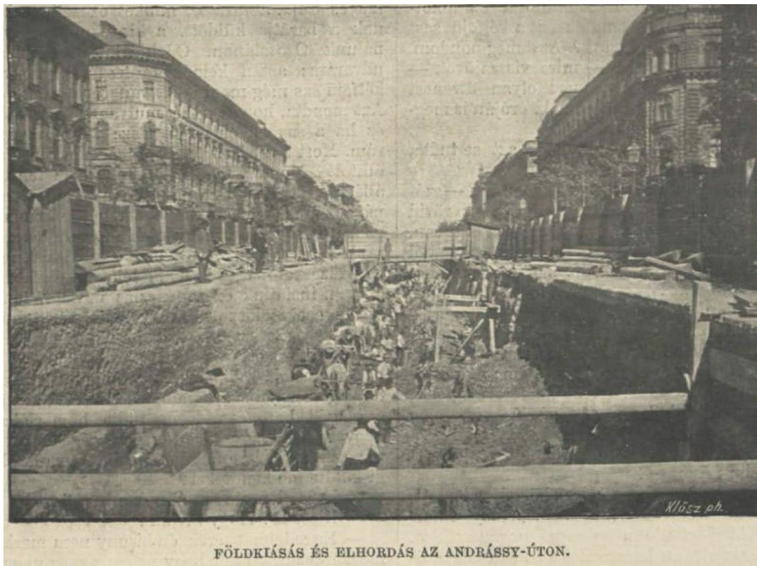
Figure 17: Construction of the Millennium Railway on Andrassy Avenue (Klősz, 1896b)
