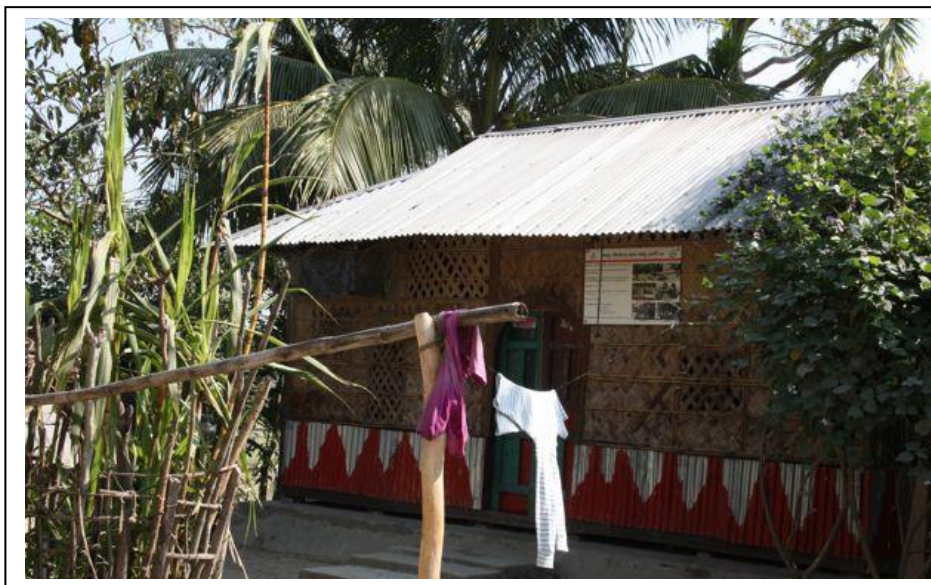
Photographs 4.6 and 4.7: Example of a home inside the embankment. This house has been supported by the NGO IUCN – it has been raised off the ground to protect from flooding, and has been reinforced with wooden plinths to protect from storm damage.
