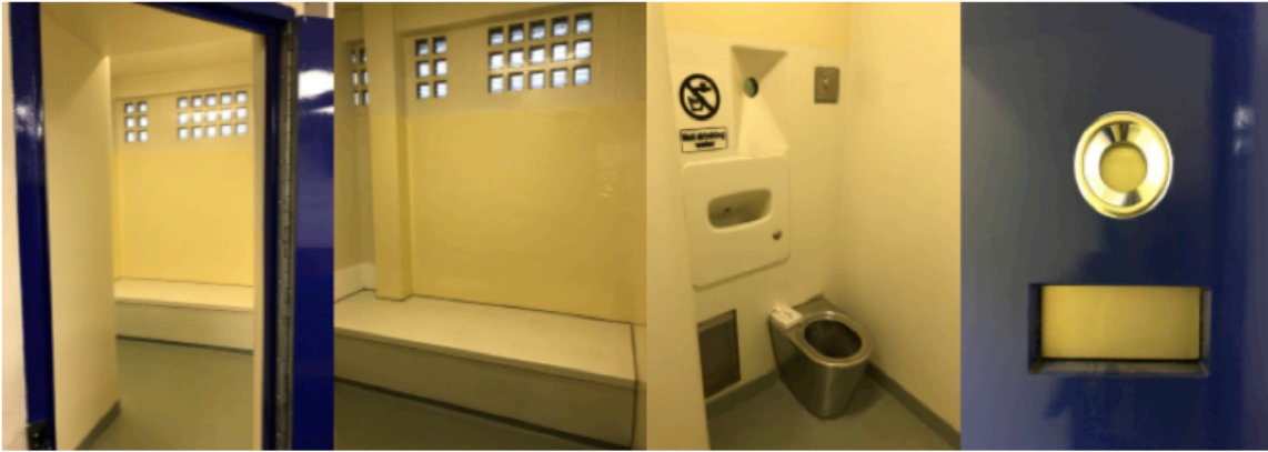
Figure 4.2 Images of an adult cell (taken on observation) showing view from door, close up of bench, washing facilities (to the left of door on entry), inside of door.
