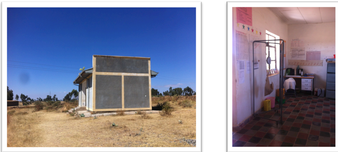
Figure 7: The exterior and interior of the health post 3
