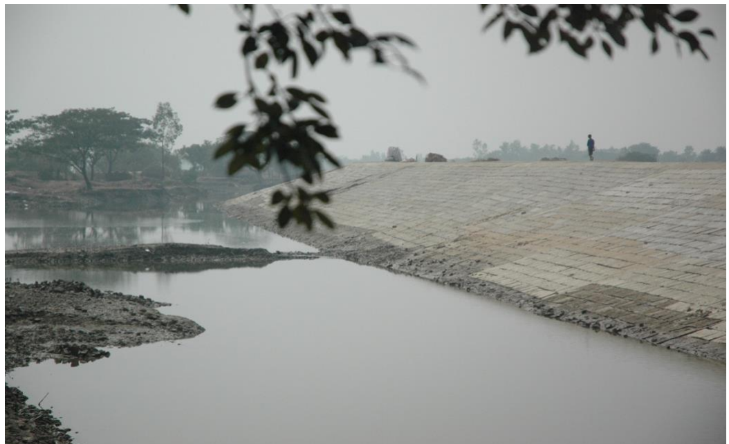
Figure 4. The construction of “modern” embankments on Bali Island began in 2016. The proposed plan is to make concrete walls for the 3500 kilometre periphery of all inhabited islands.
