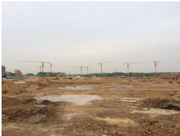
Figure 4.1 A view of the construction site
