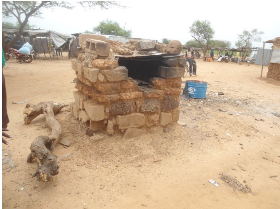
Figure C.2: Example of fixed outdoor cookstove, self-built by a refugee household in Goudoubo. Source: Practical Action, Moving Energy Initiative.
