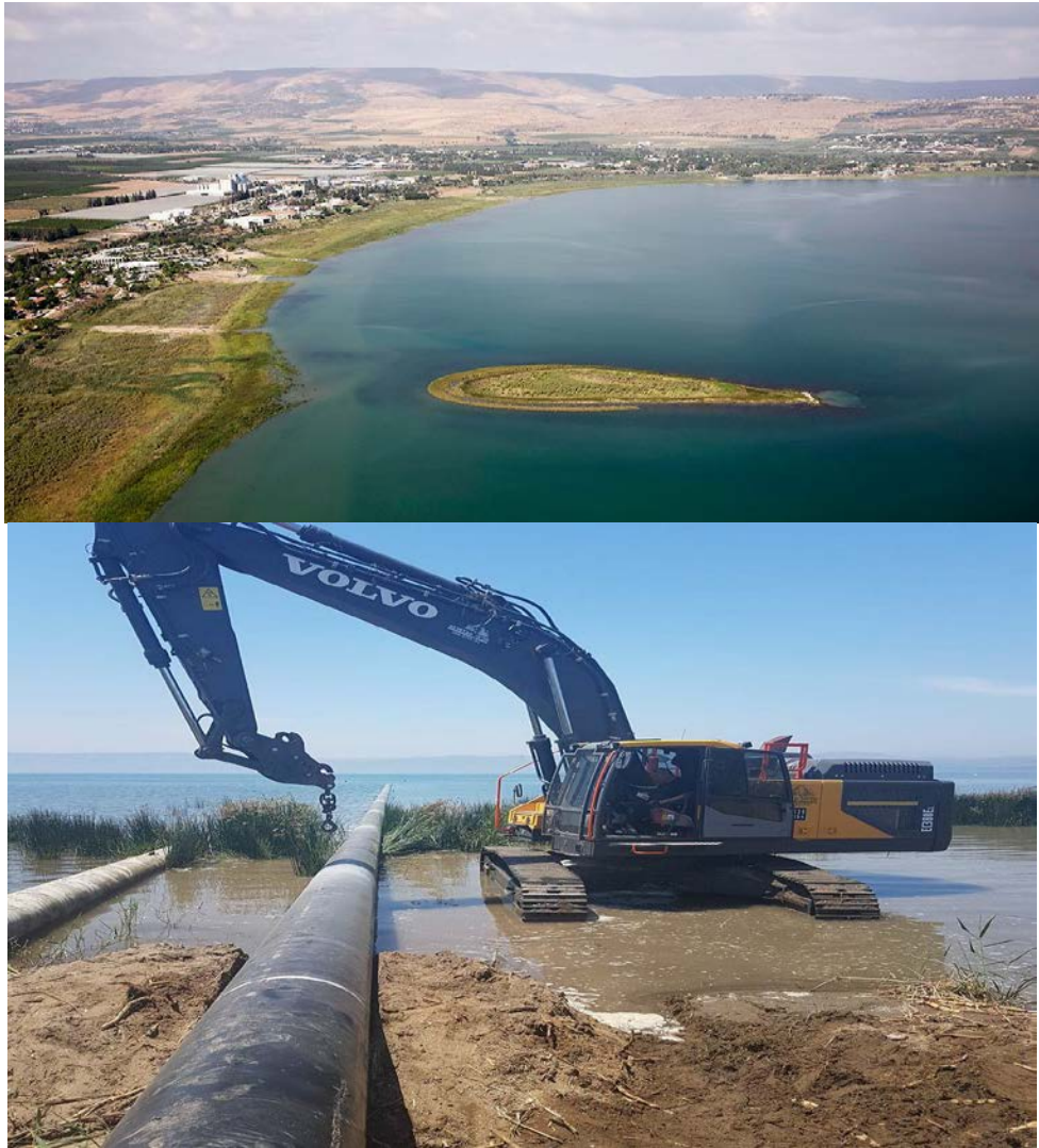
Figure 5.25 the expanding island in the Lake Tiberias (above), and Mekorot's pipelines being installed to alleviate the water drop (Ynetnews, 2018)
