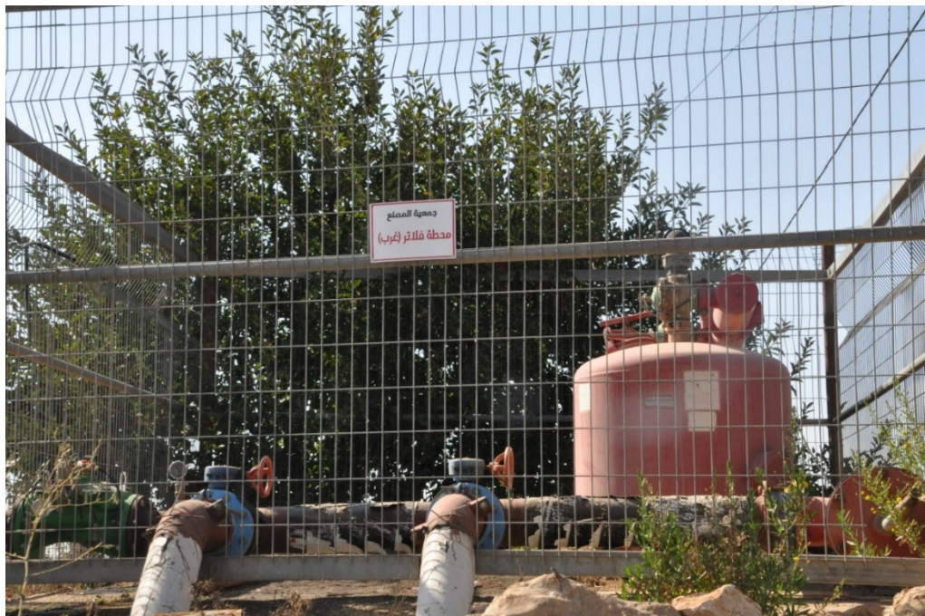
Figure 7.9 Filtering station belonging to one of the cooperatives, Al Masna' (Author's photo, 2016)
