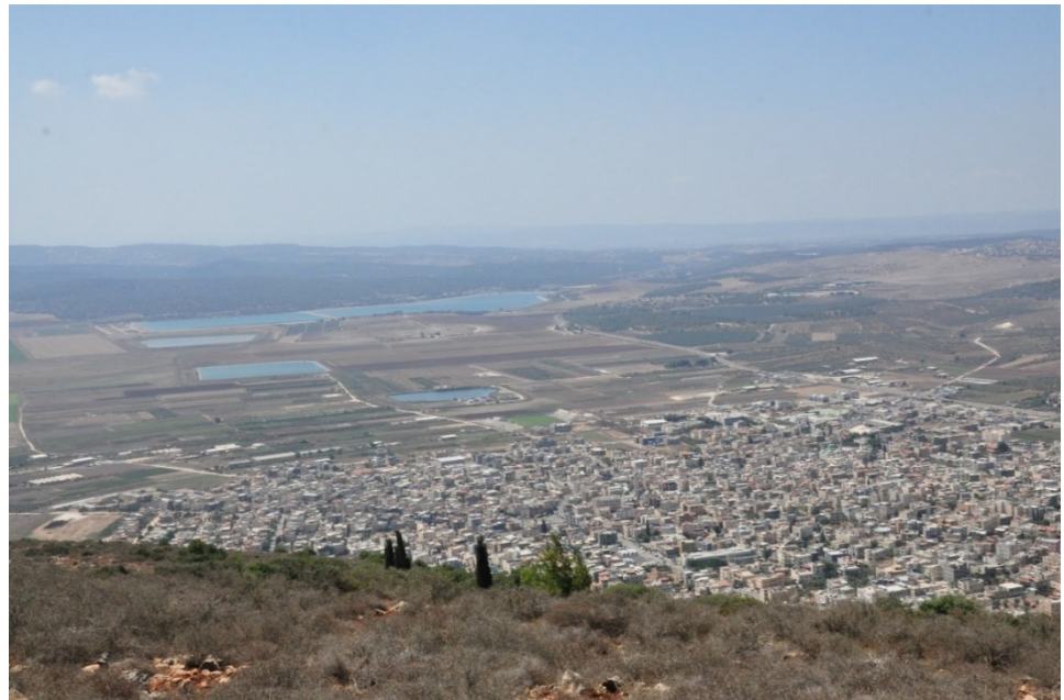
Figure 5.3 A recent picture of the Eshkol reservoir plant, facing Kufr Manda village (below) (Author's pictures, September 2017)
