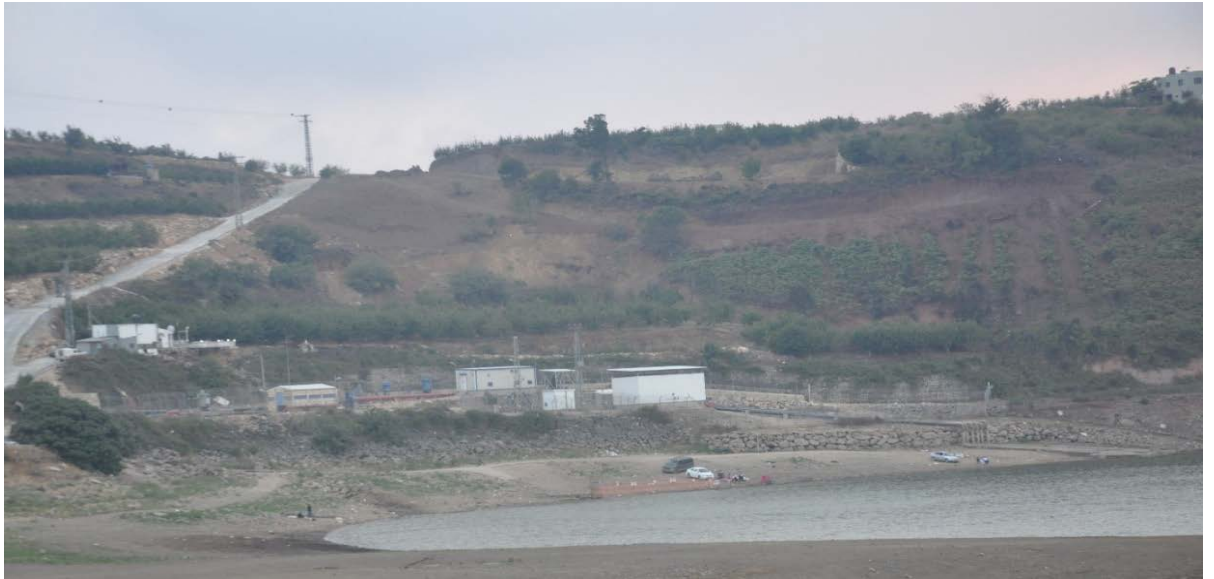
Figure 6.18 Mekorot's pumping station on Birket Ram (Author's picture, December 2016)
