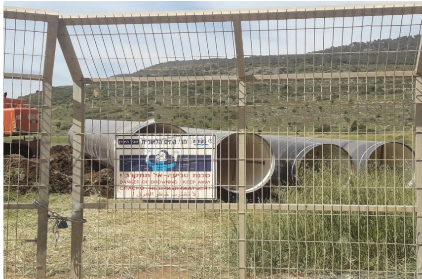
Figure 5.24 the pipes laid down by Mekorot in Al-Battuf, inside the fenced area of the NWC canal (Alarab news agency, 2018)
