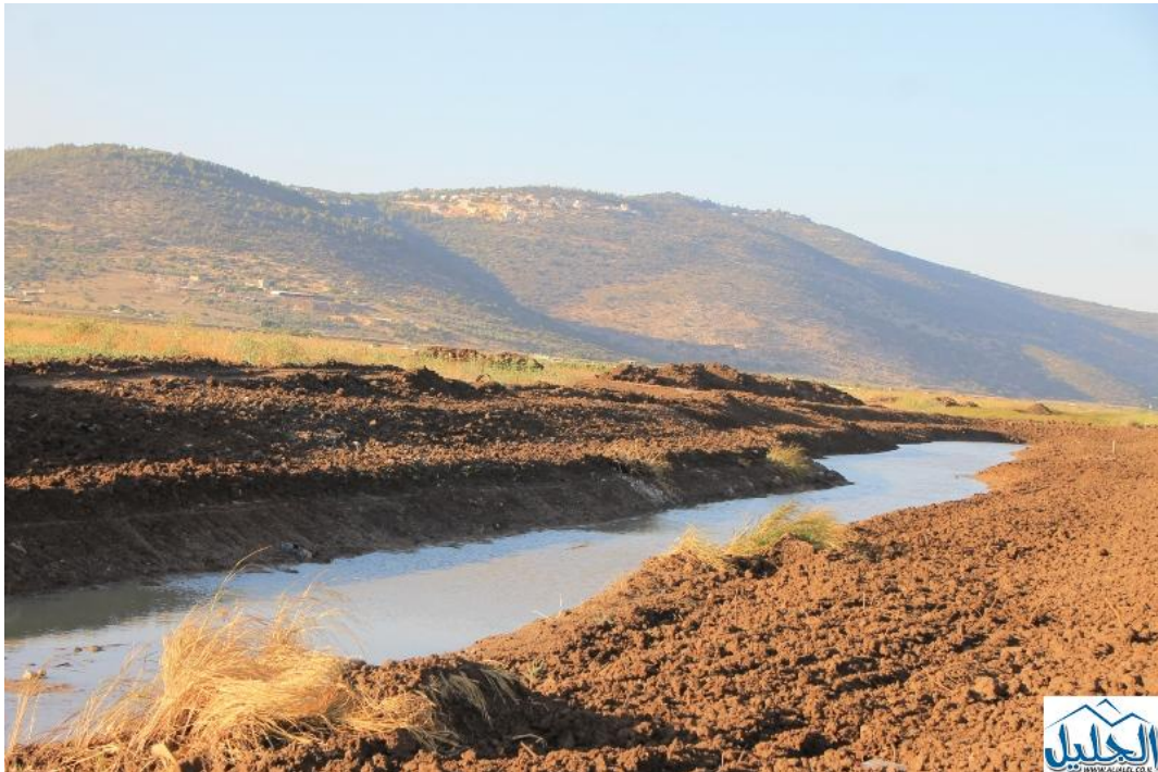
Figure 5.23 Resumed work on the zero Canal by the River Drainage Authority (Al Jalel, 2018)
