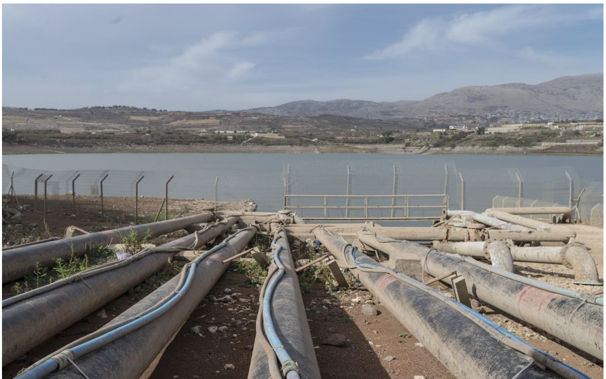
Figure 6.19 Mekorot's pipelines pumping water from the Lake to Israeli settlements (Al-Marsad, n.d.)
