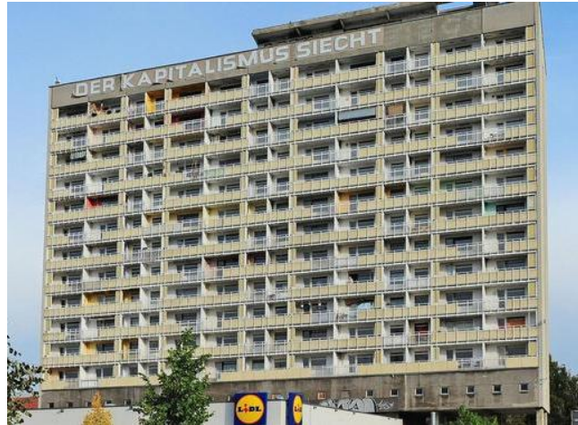
Figure 40: The same building in 2015 with a new slogan illegally installed saying “Capitalism is ailing” (photo by Anja Schneider, Dresdner Neueste Nachrichten , screenshot by the author).
