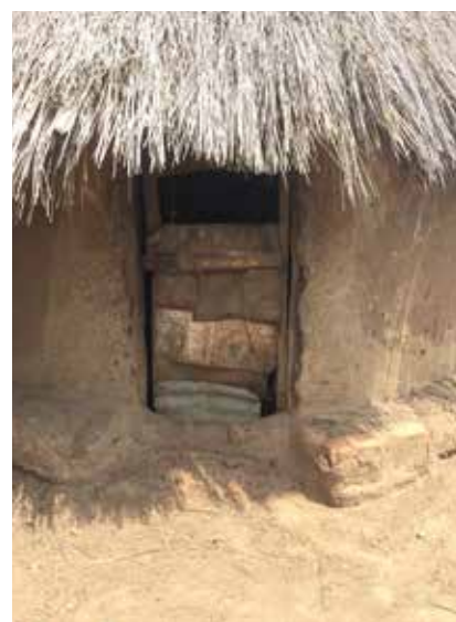
Figure 2.4 Hut with a door made of WFP tins, Pabbo Memorial site.
