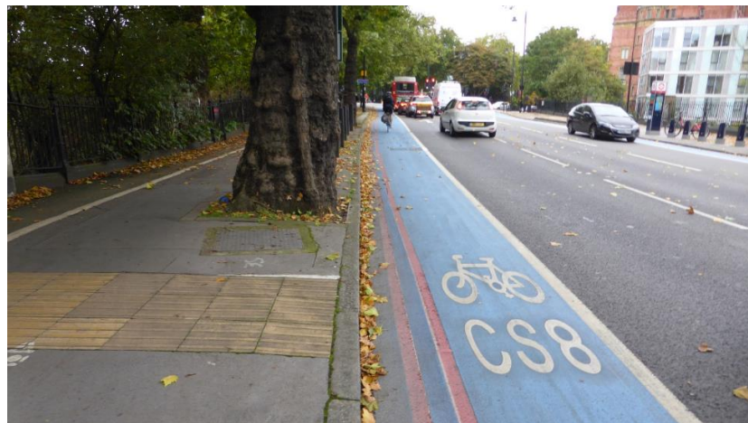
Figure 2.A.2: Cycle Superhighway 8 - Opened in 2011 - Painted lane
