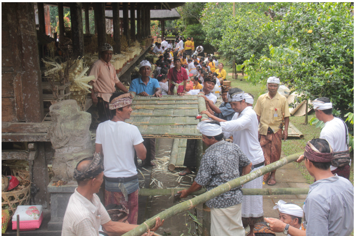
Fig 6.24: Men at work sculpting bamboo into scaffolding for the offering towers ( sanggar agung ). Photo credit: I Made Ari Yudiana
