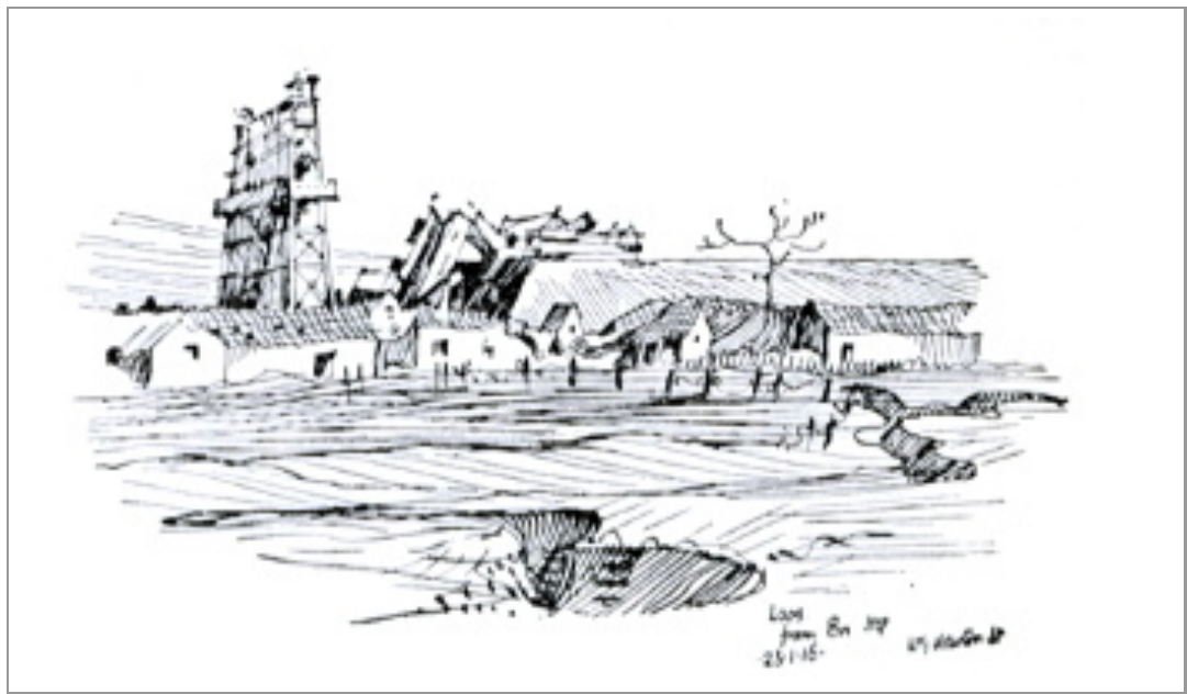
Figure 49 - Loos showing the 'Tower Bridge' winding gear tower 431
