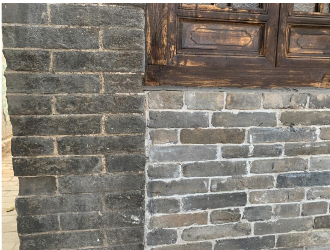
Figure 5-5. The contrast between the old bricks made in the Qing Dynasty and the new bricks used in the restoration (Source: author, 2021).
