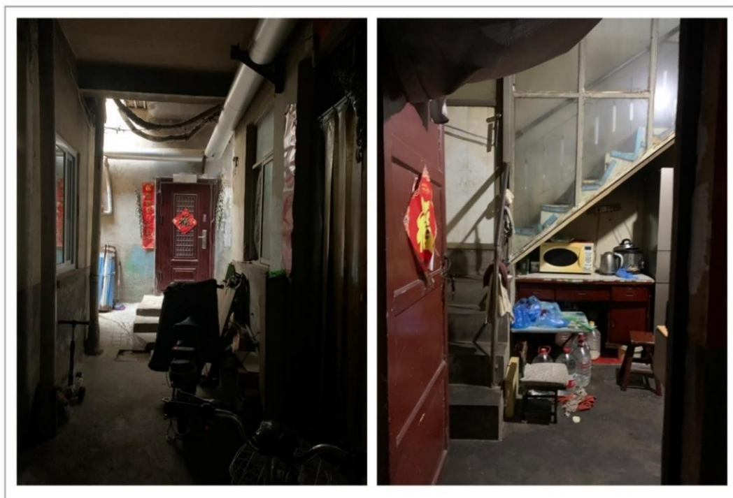
Figure 4-12. The hallway (left) and the kitchen (right) of a house in Cangxiang Street Historic District (Source: author, 2021).
