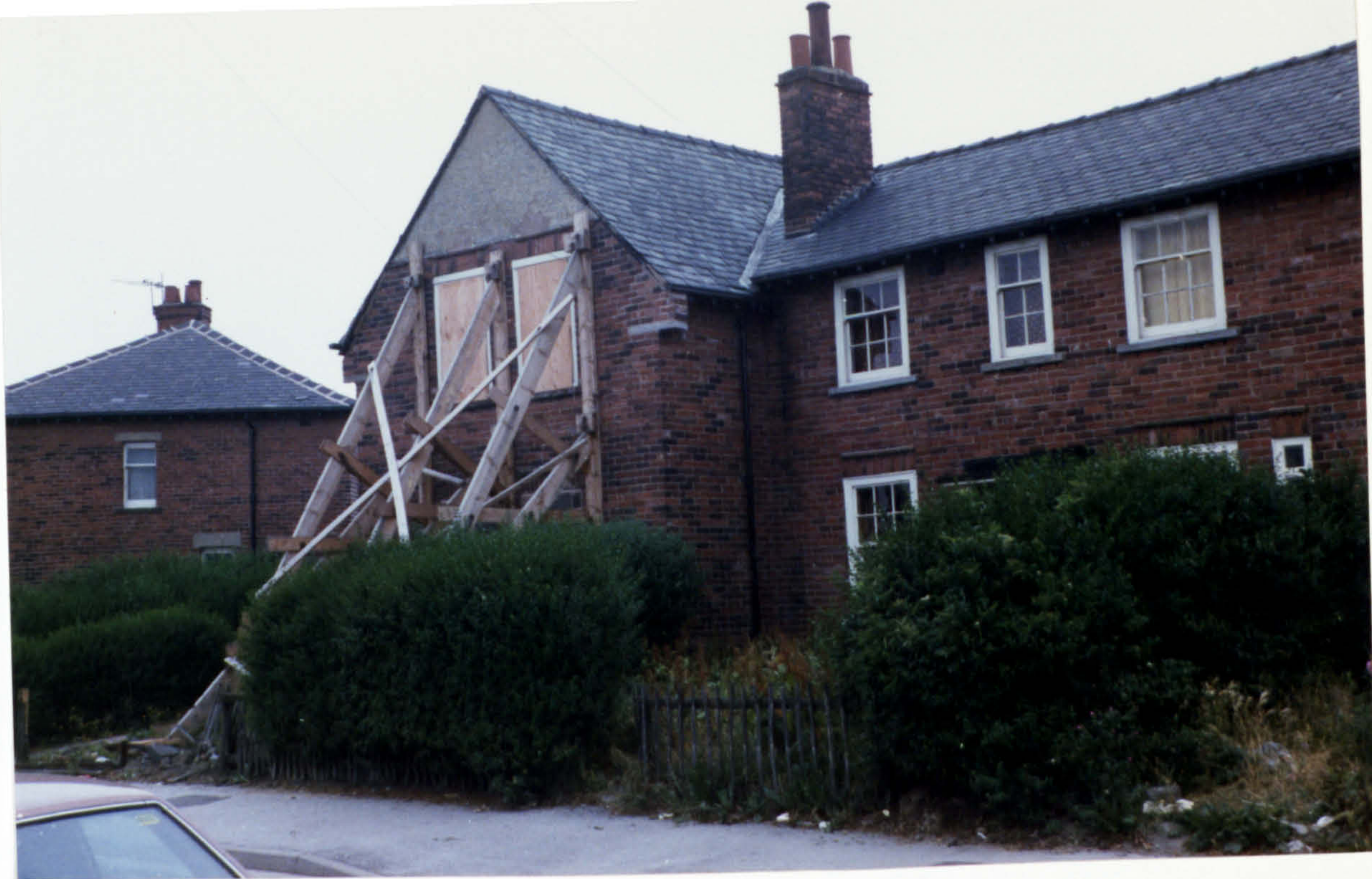
10. A large but decayed northern cottage estate suffers from wall-tie failure and is under threat of demolition.
