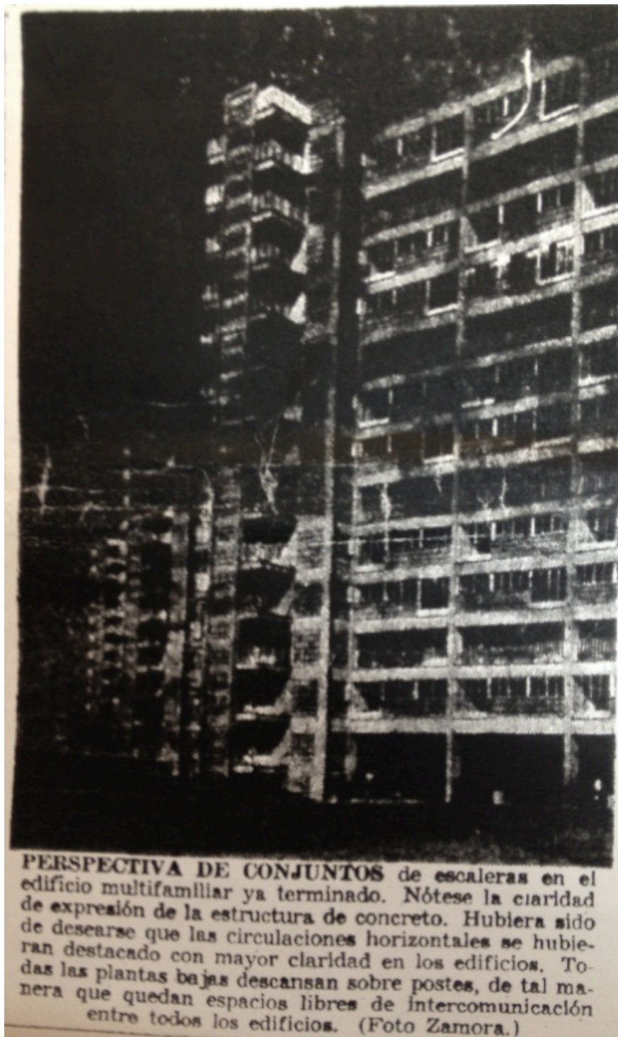
Figure 5.20: Photograph of a stairwell at the CUPA, newspaper clipping from the inauguration of the CUPA, 2 September 1949. Caption reads: 'Notice the clarity of expression in the concrete structure'. Source: Excelsior , 4 September 1949, third section, p.10.
