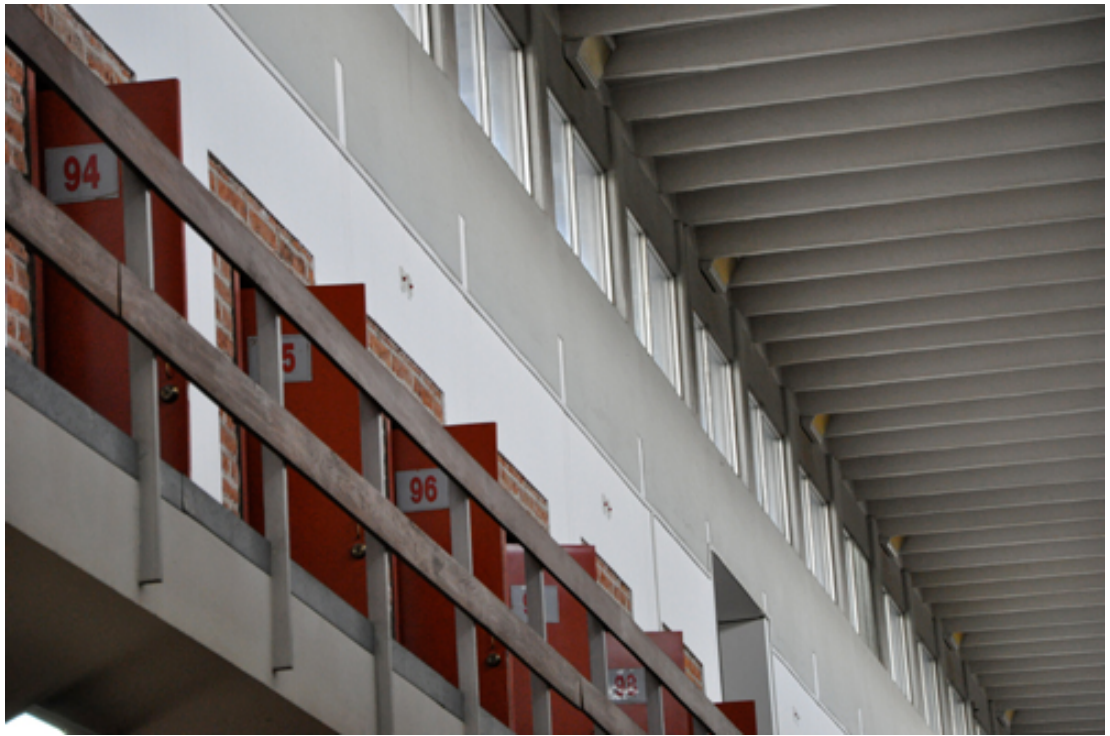
Figure 2.6: Detail of the old prison cell doors, currently housing the Presidential Archives of Mexico, Archivo General de la Nación, Mexico City. Source: Photo by Author. April 2010.
