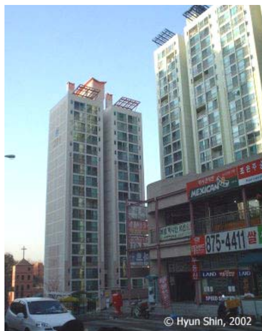
Figure 8-1: View of KNHC-provided public rental flats
