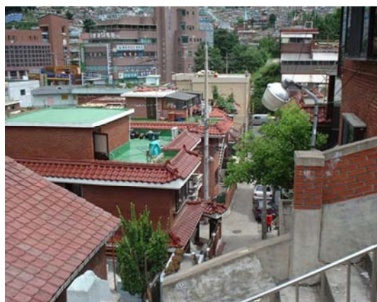
The picture below shows examples of multi-dwelling houses near Nangok neighbourhood, one of which has a roof-top extension.
