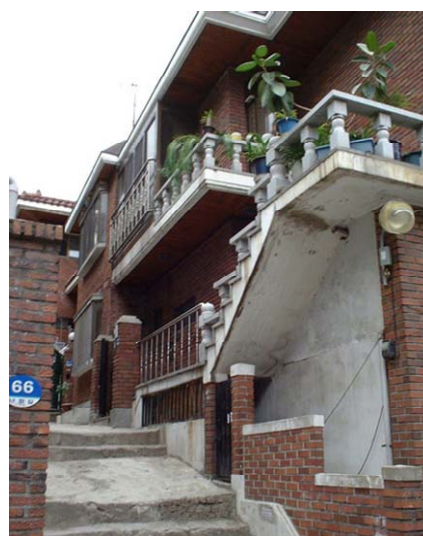
The picture above shows a lateral façade of a multi-dwelling house. Each door in the picture leads to a separate sub-divided accommodation. The door in the lowest floor leads to a semi-basement dwelling.
