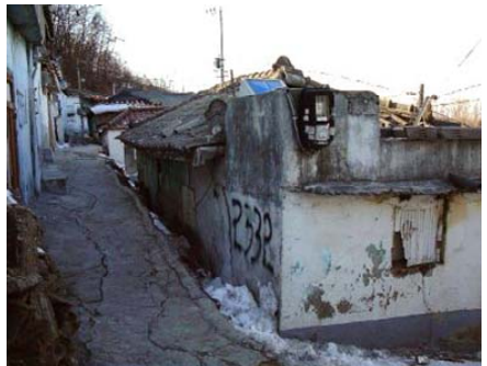
(e) Rear wall of the house on the right lower than road surface. No sun light through rear window
