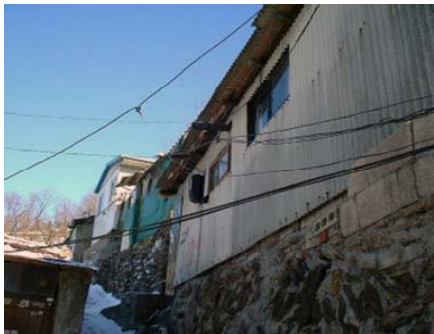
(c) Exterior wall of a house covered with slate sheets. Elevated foundation due to the slope
