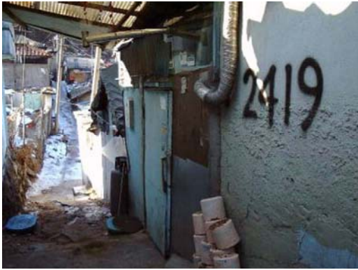
Point A. Exterior view. Exhausted briquettes are stacked against the wall. The number '2419' is a dwelling identification number attributed by the developer.
