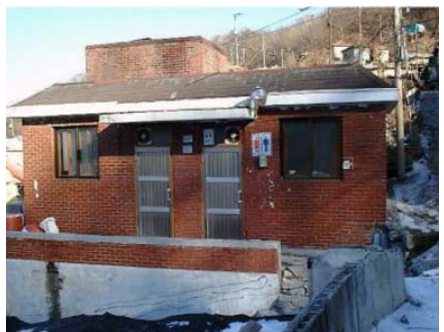
(f) View of public toilets provided and managed by the local authority.
