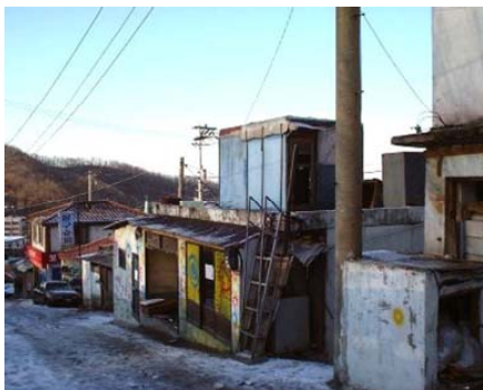
(g) Roof-top extension along the main thoroughfare
